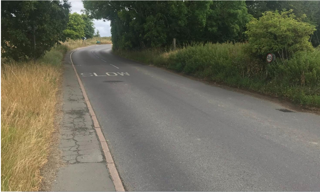
Figure 3.2: Existing School Road Footway (Looking North)
