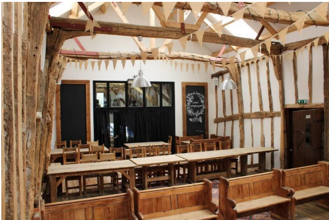
Pannington Hall (Jimmy's Farm): Main barn interior
