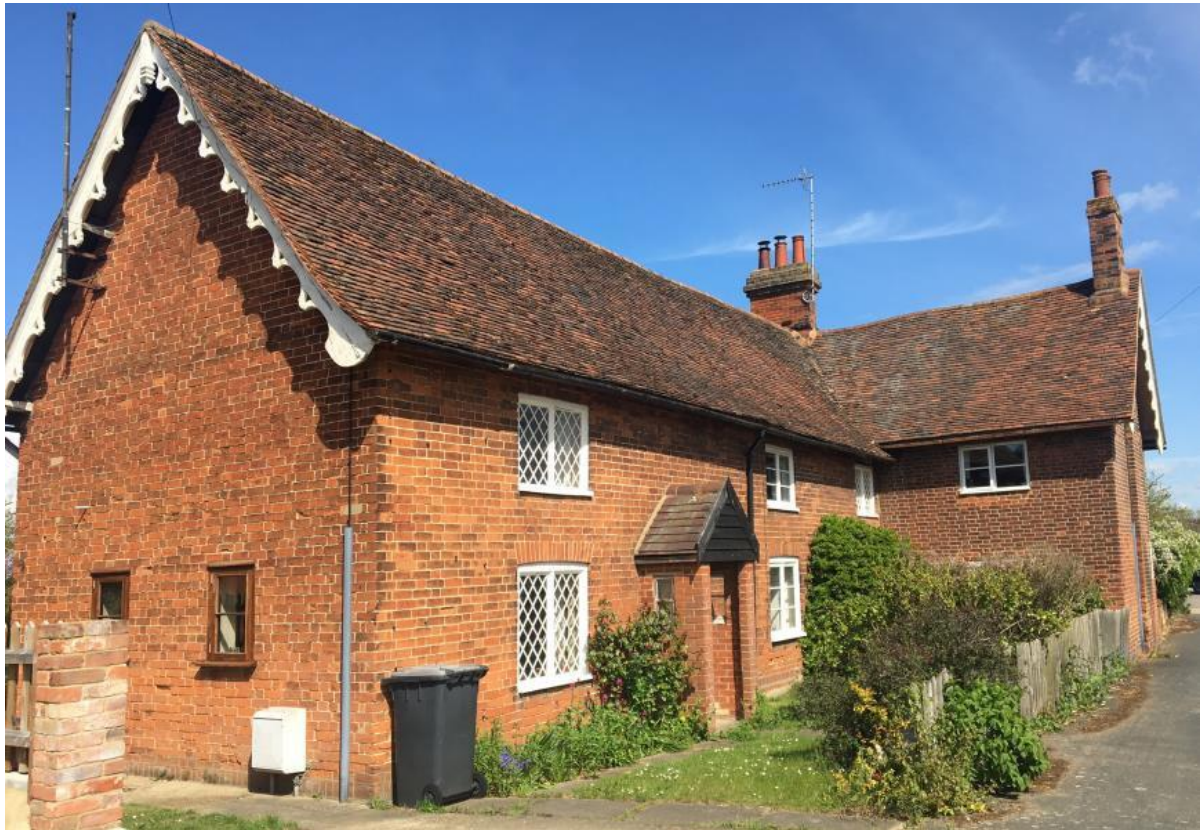
1-3 Ostrich (Bourne) Cottages from the south-east.
