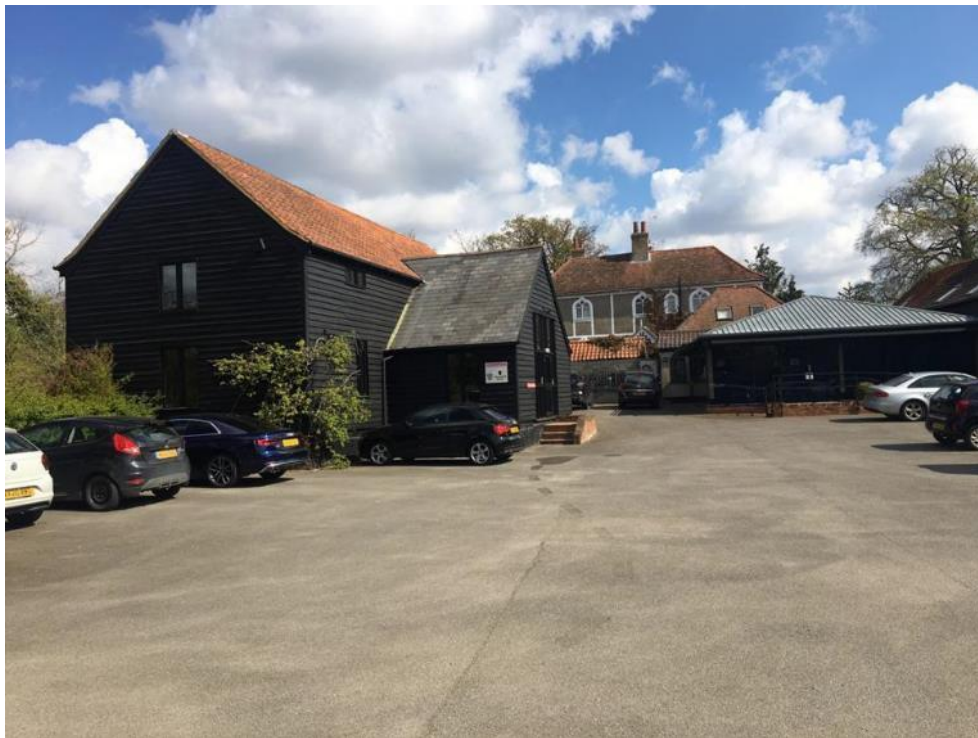
Unit 2 Peninsula Business Centre from the east (facing the courtyard) with the modern unit 3A top right and Listed farmhouse (Park Farm) to north.
