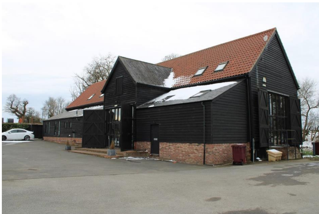
Unit 1 Peninsula Business Centre from the east (facing the courtyard)
