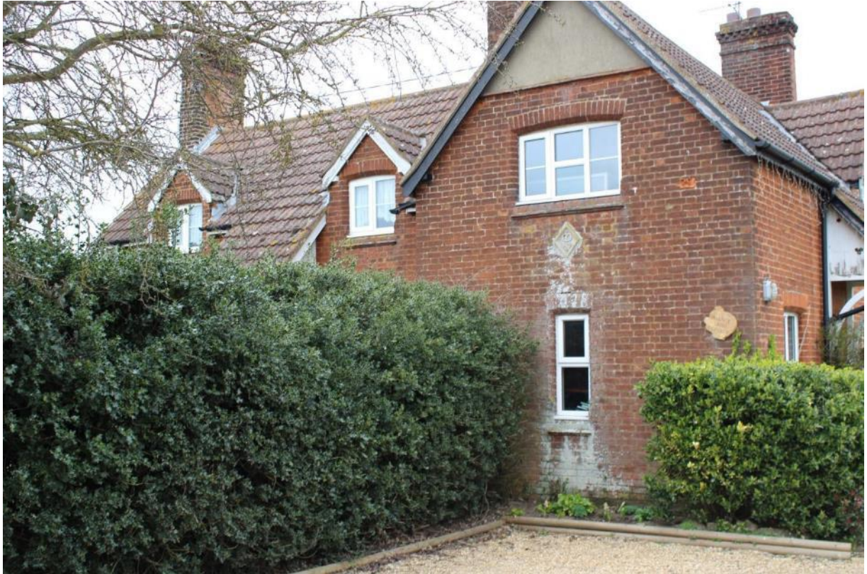
Walnuttree Cottage south gable with date plaque.
