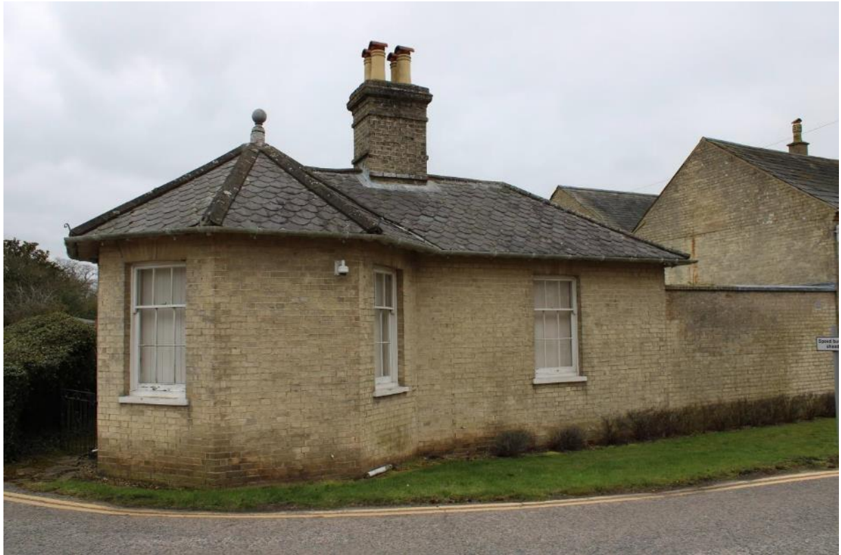
The Mansion Stable Block lodge.
