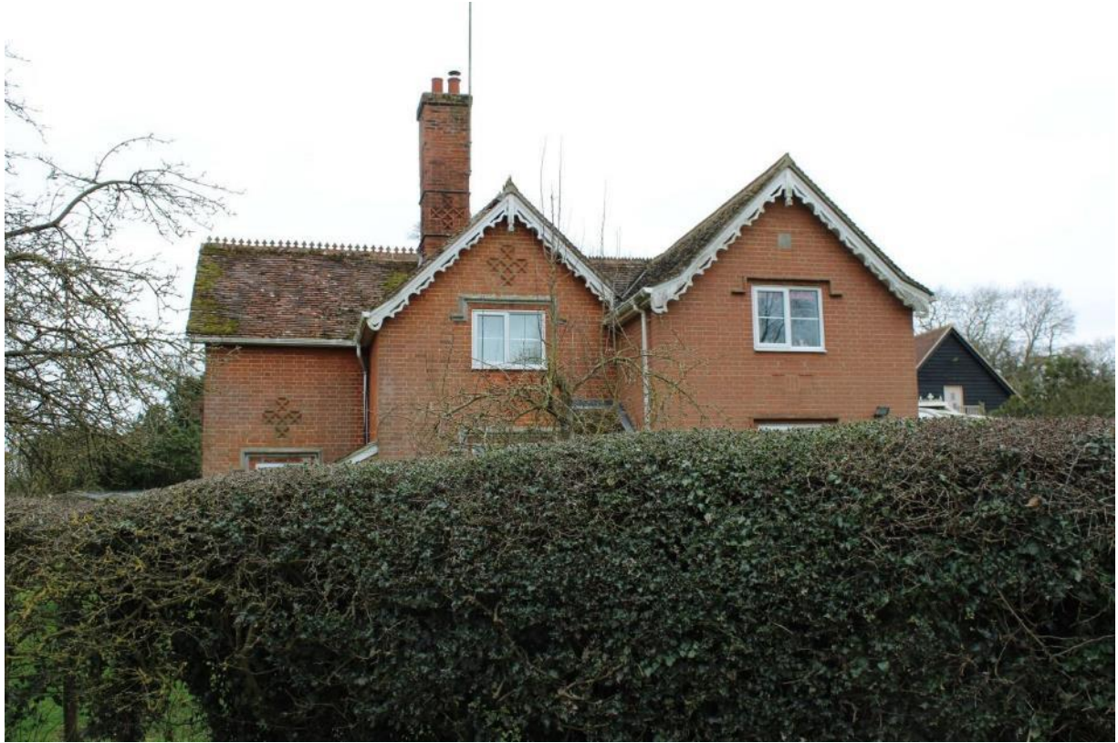
Pannington Hall Cottages From the east.
