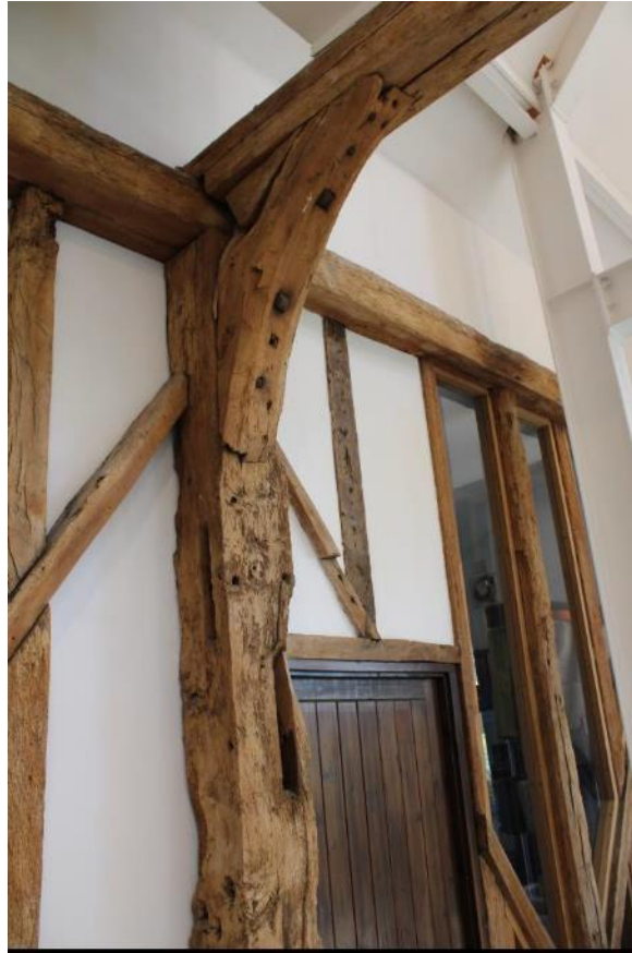
Unit 1 Peninsula Business Centre interior
