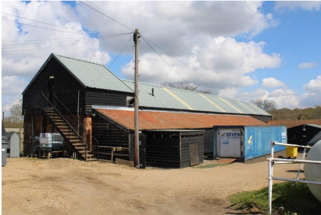
Pannington Hall (Jimmy's Farm): Main barn from south-east with later additions.
