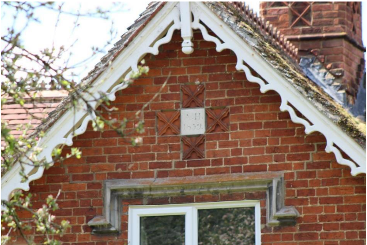
Pannington Hall Cottages: north-west gable showing date plaque, hood mould decorative brick insets, roof and ornamental ridge tiles and barge boards,
