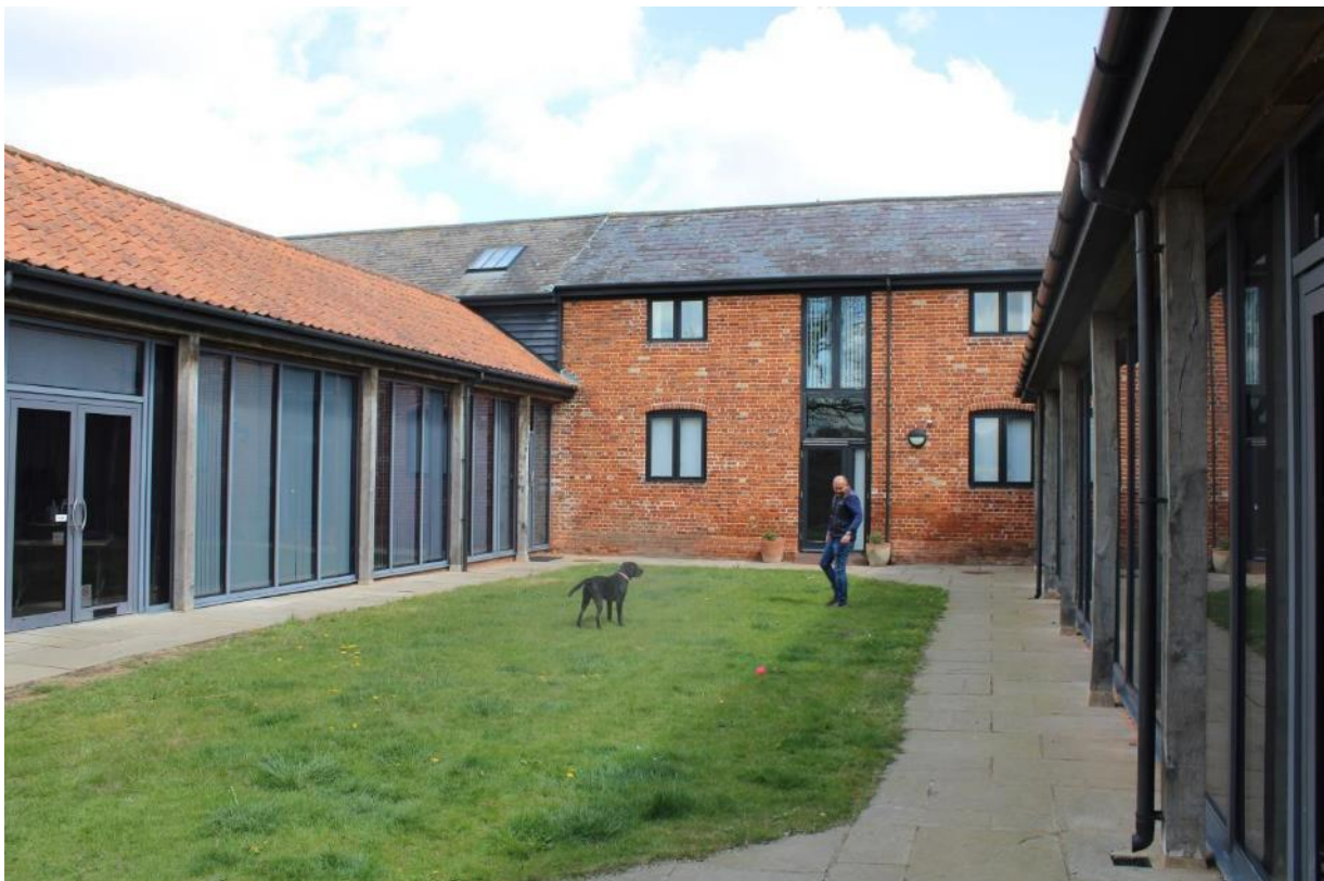
Unit 5 Alton Business Centre (Valley Farm barns): south-west elevation with Unit 4, to left, and 5a, to right, with courtyard between.
