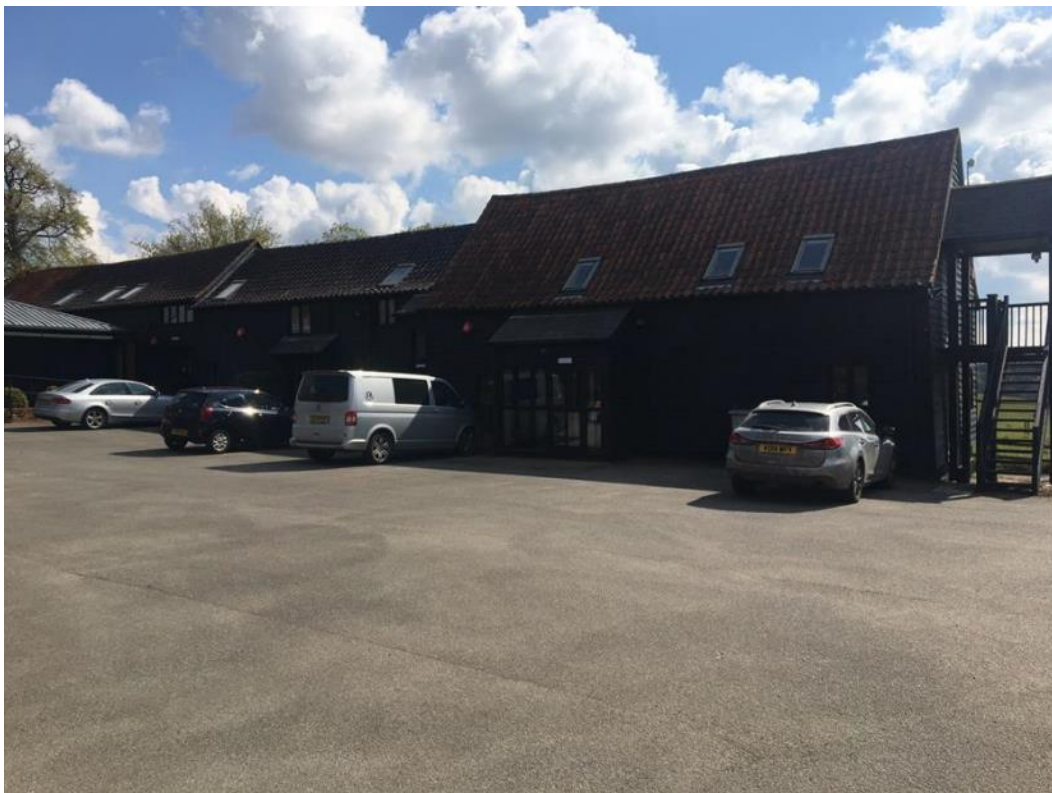
Units 3-5 (left to right) Peninsula Business Centre. West elevation facing the courtyard.
