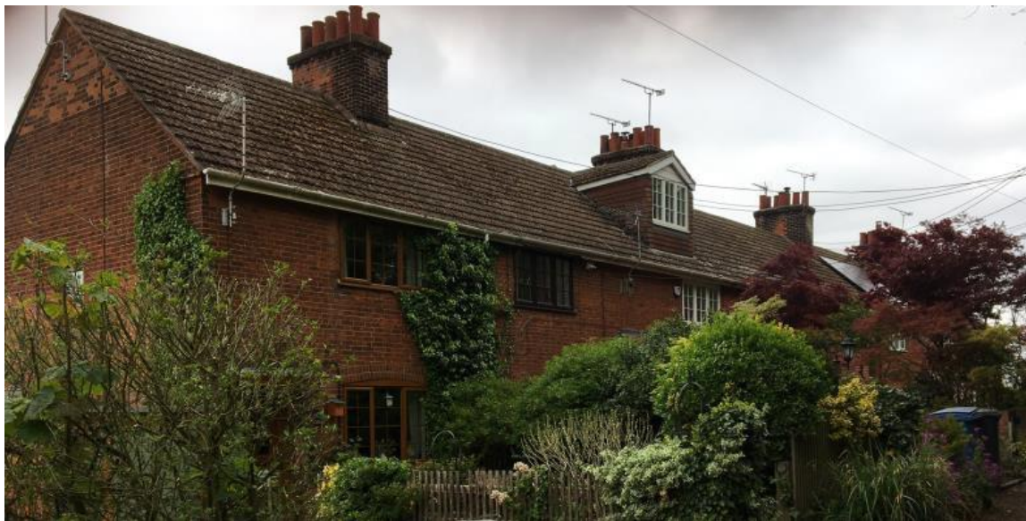
Bourne Terrace from the south-west.
