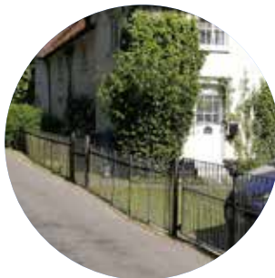
Metal rail fencing
