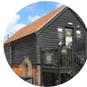
Timber framed barn
