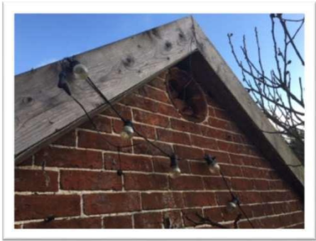
Period brickwork and oak fascia
