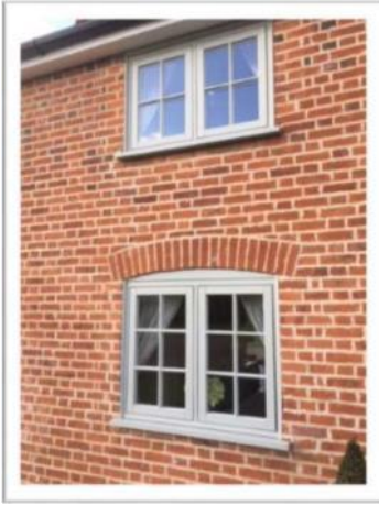
Period brickwork and window arch
