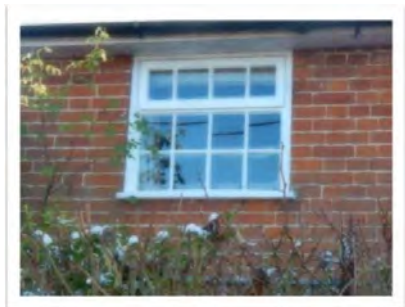
New build brick work and plastic downpipe
