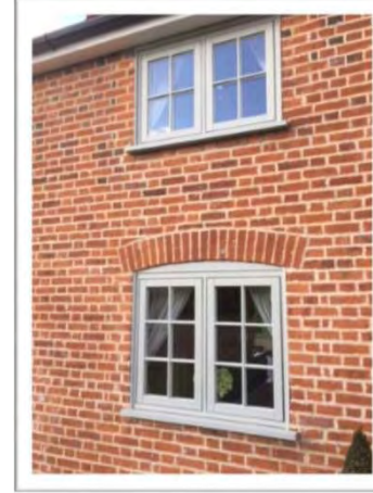
Period brickwork and window arch
