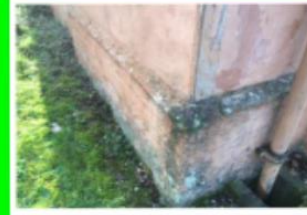
Corner brick foundations and render
