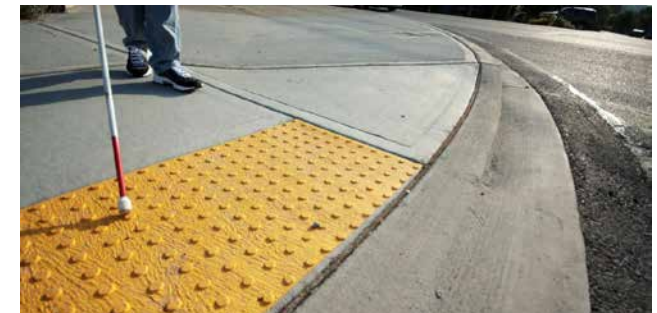
Figure 48: Example of tactile paving to facilitate movement for people with visual impairment.
