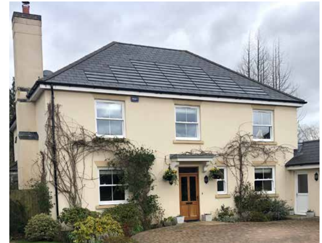
Figure 52: Use of shingle-like solar panels on a slate roof, with the design and colour of the solar panels matching those of the adjacent slate tiles.
