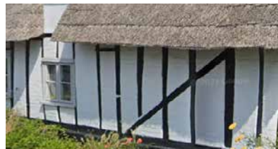
Render with Tudor style timber framing
