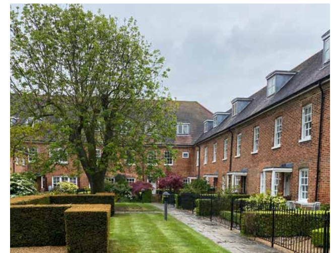
Figure 50: Positive example of properties with small front gardens overlooking the adjacent open space, Tattingstone.
