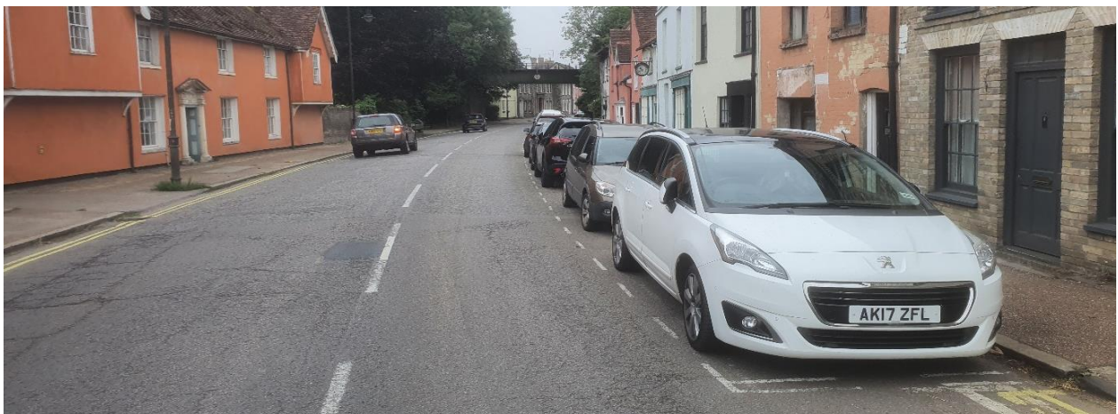
Figure 2 – Example of on-street parking location limited waiting could be implemented
