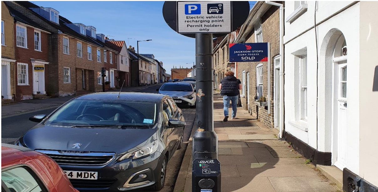
Figure 16 – Example of an on-street electric vehicle charging point
