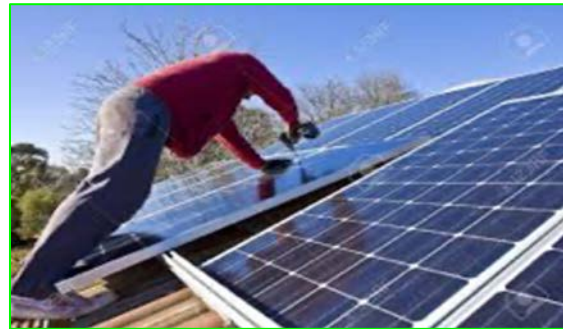
Installing solar panels
