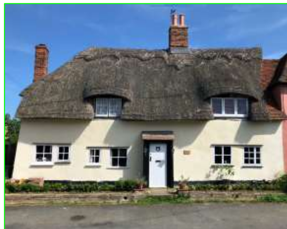
17 th -18 th Century timber frame house
