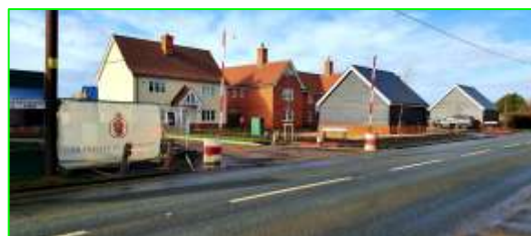
Red House Farm development
