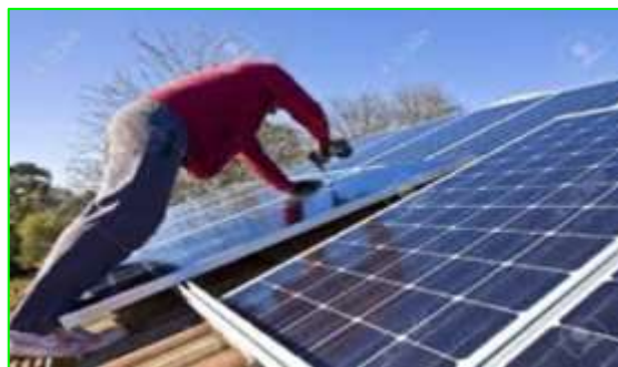
Installing solar panels
