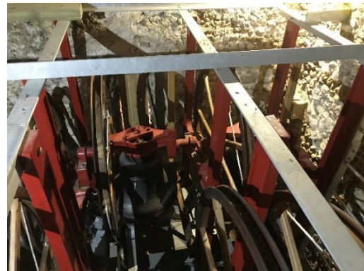
The new bell frame and bells
