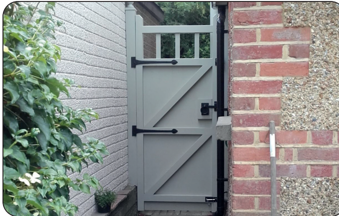
Access gate to back gardens, that provides a clear route for refuse bins to be moved from back gardens to the front of the property for collection
