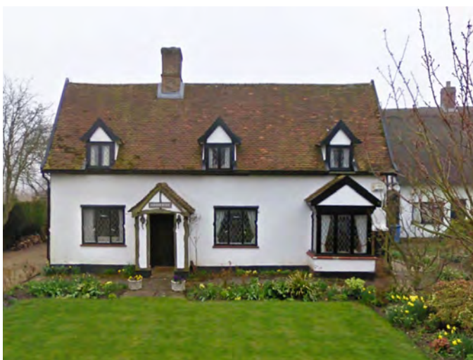
Figure 16: Post office, Grade II Listed Building.
