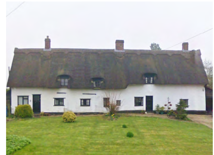
Figure 22: Traditional thatched roof building.
