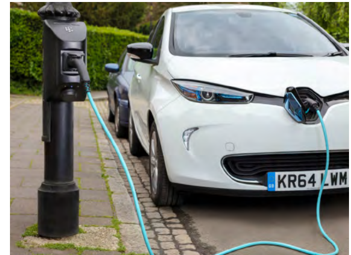
Figure 45: Public car charging point incorporated into the street design.
