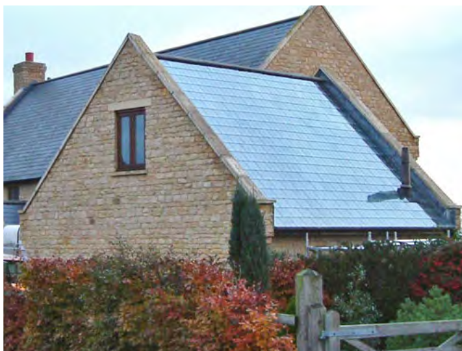
Figure 39: Retrofitted solar panels integrated sympathetically with a traditional building.
