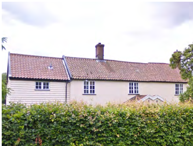
Figure 23: Dwelling with pantile roof tiles.
