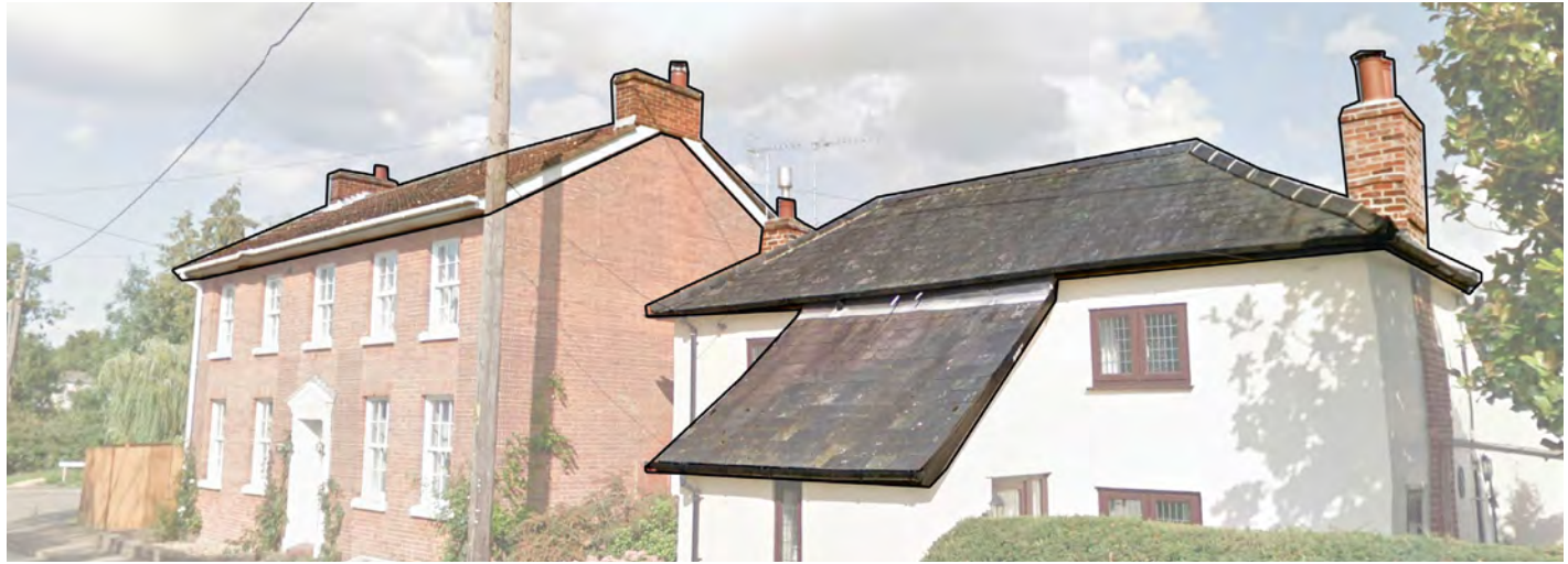
Figure 20: Varied roof line along Bury Road at the northern edge of the Main Population Hub.
