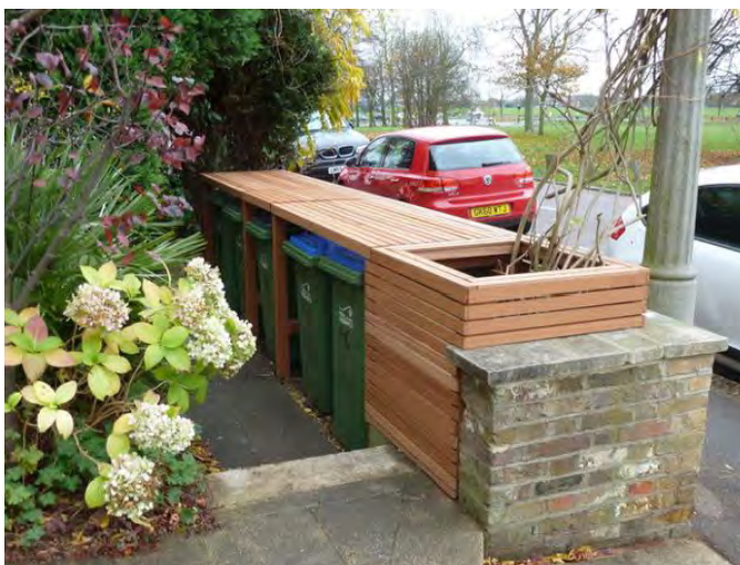
Figure 47: Waste bin storage used as a boundary treatment.
