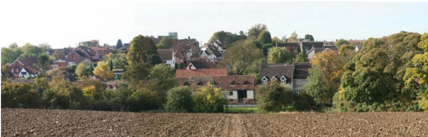
View from footpath east of Lower Road
