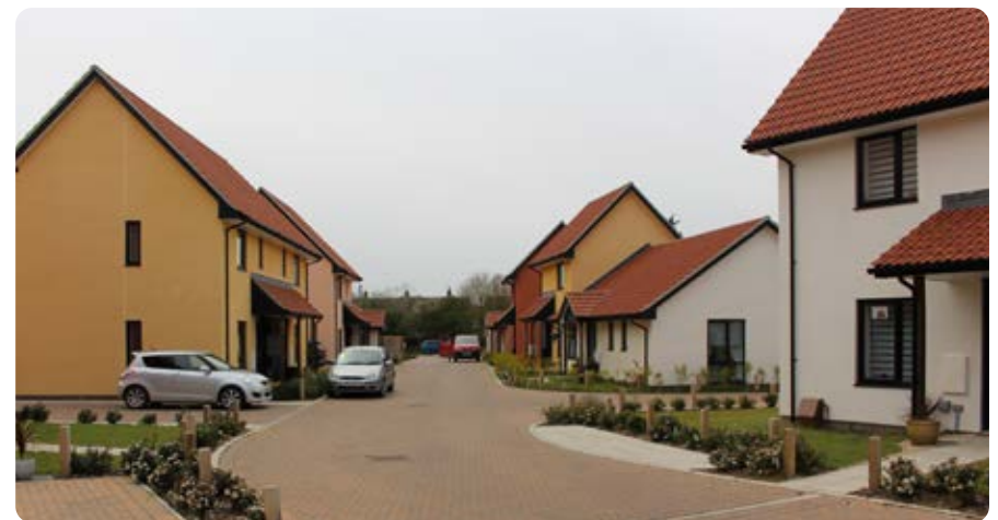
View to Peek Close - a well designed community led affordable housing scheme
