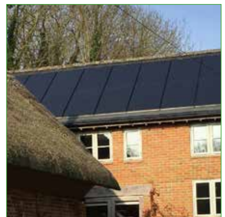
A solar PV array integrated into the slate roof. Image © Historic England
