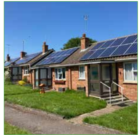
Solar PV panels, Lavenham
