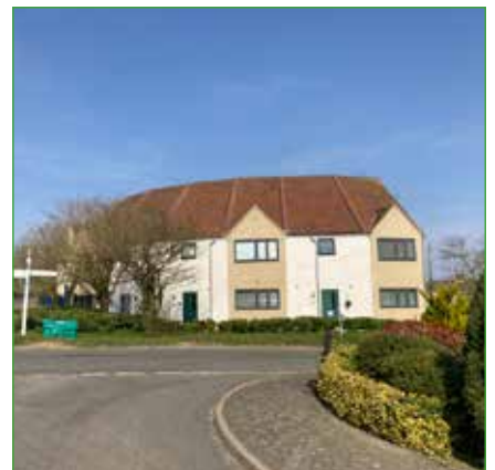
Poorly proportioned elevations with overbearing curved roof line
