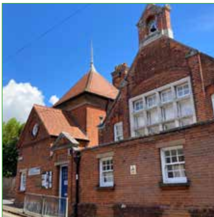
Primary School: a varied roofscape.
