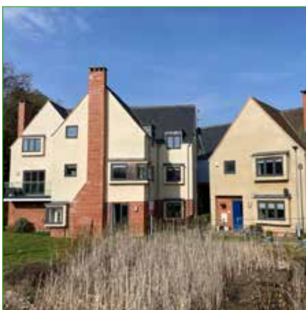
Old Station Close
