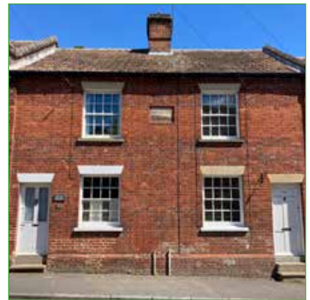
< The simple elevations of these homes display with a pleasing variety of complementary materials. Brick façade with contrasting pale opening surrounds and projecting horizontal band contrast with a simple off-white painted render.
