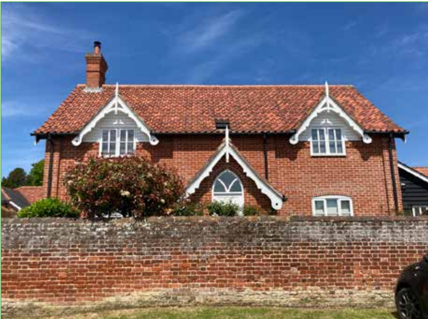
An attractive building and boundary wall constructed in brick.
