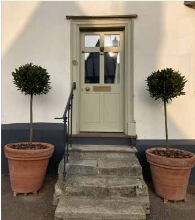
High quality timber doors with simple high quality detailing
