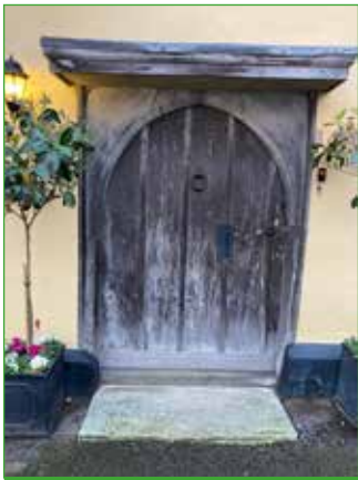
Traditional timber door.
