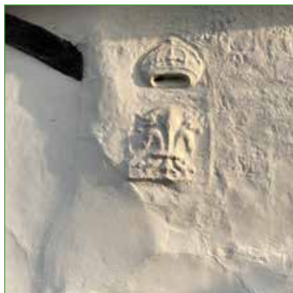
Plaster pargeting to facades
