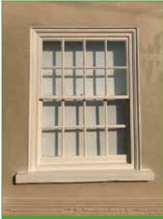
Traditional timber sash windows with ornate moulded linings.
