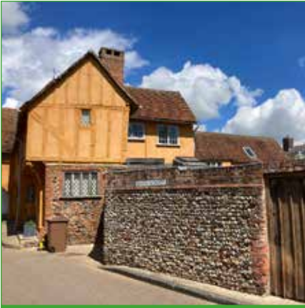
Barn St: Traditional flint and brick wall.
