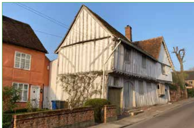
The Priory, Lavenham
