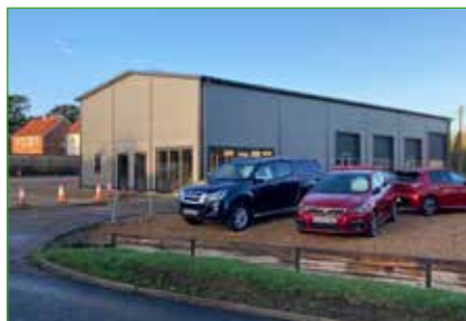
New Garage on Sudbury Road
