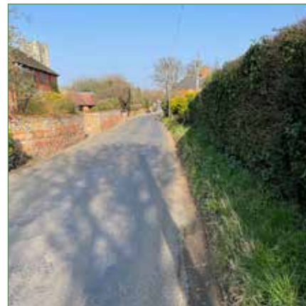
Bridge Street Road, a narrow highway which does not benefit from a footway
