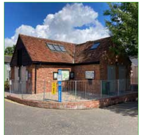
Public toilets, Cock Horse Inn Car Park
