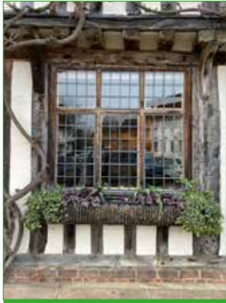
Traditional timber window.
