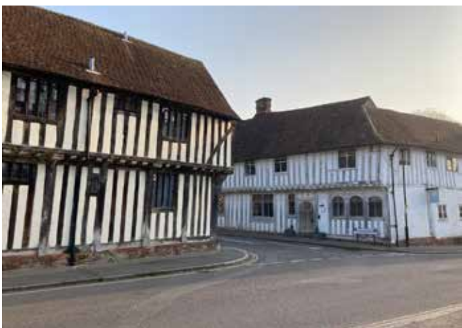
Corner of Water Street and Lady Street
