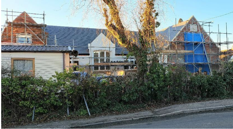
Figure 47: School House under renovation.
