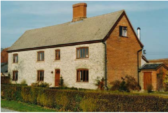
Figure 44: 16th century farmhouse encased in brick in the C19th, and roof tiled.
