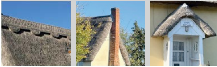
Figure 24: thatched roofs in Hitcham.
