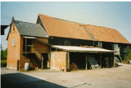
Figure 43: Timber-clad and weatherboarded barn. Originally built C1 as stables converted into barn 1800s and Granary added.
