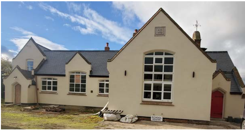
Figure 48: Old School House completed.
