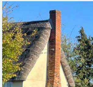
Chimney at gable end
