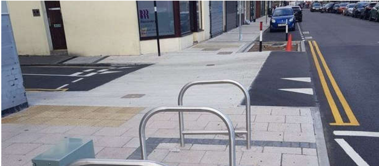
Figure 22 – Example of a continuous footway
