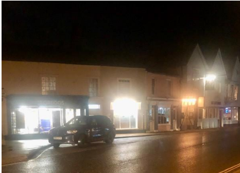
Greggs, The Spice takeaway, and the George Inn at night. Greggs has no external illumination using its well lit interior to invite customers in, whilst The Spice and The George use external down lighters.
