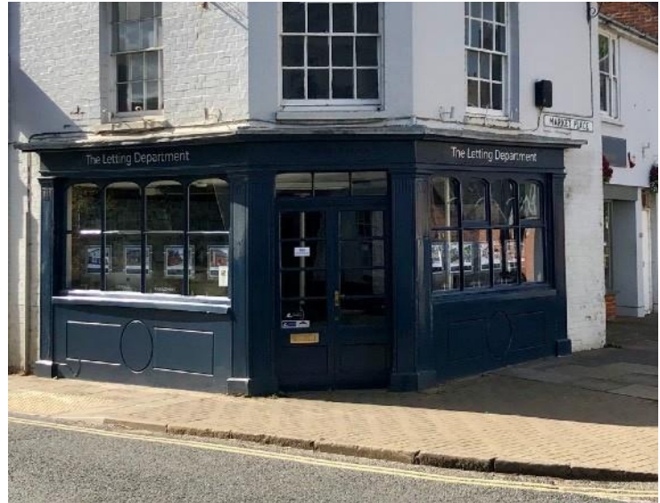
No. 1 Market Place Grade II [originally part of 37 & 39 High Street] circa 1840. Whilst a modern shopfront it incorporates traditional features of pilasters, decorative stall risers, vertically divided display windows with flat rounded heads.
