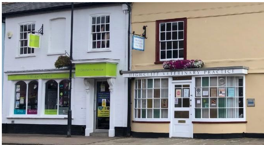
Nos 96 & 98, Grade II, Mid Victorian. The veterinary practice at 96 has a wood shop front with a small glass pane double bay window and central door, The shop at 98 has display window equally divided with central pilaster to reflect the spacing of the upper floor windows. The doorway is separated with its doorcase pilasters and deep set, corniced and flat roofed door hood.
