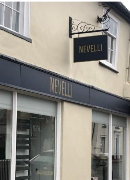
A simple painted fascia and matching hanging sign with on ornate decorative bracket.
