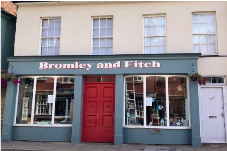
No. 50 Grade II, C16-C17 build with late C18 front. Ground floor displays a C19 Double bay shop front contained within traditional pilaster and fascia surrounds.
