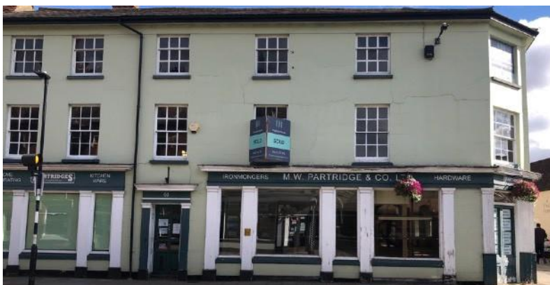
No 60 Grade II, Probably C18. Shopfront wraps around this corner property with an entrance door in wood case with fluted pilasters on the corner all with Doric pilasters and continuous entablature.
