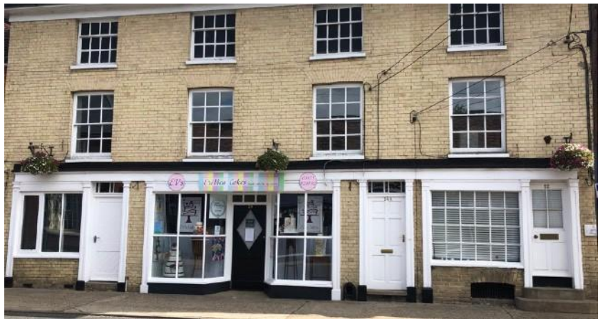
Nos 22 to 26 Grade II Early Victorian, The floor shop fronts and entrances with pilasters display a variety of traditional designs and which are unified under a continuous entablature.
