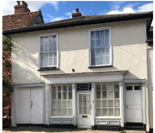
No. 9 Grade II, Late C18 to C19. An old timber shopfront probably inserted in Victorian period in a Georgian style with small glazed panes decorated stall risers, central timber and 6 pane door with transom fanlight over.
