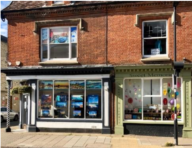
No. 1 Market Place Grade II [originally part of 37 & 39 High Street] circa 1840. Whilst a modern shopfront it incorporates traditional features of pilasters, decorative stall risers, vertically divided display windows with flat rounded heads.
