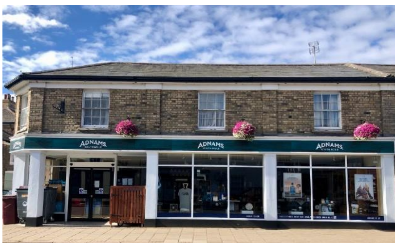
No 73-77 Grade II Built in 1834 as part of the planned Queen Street development. The shopfront is modern but note it retains the outline of the three original units by reflecting the upper storey projecting brick pilasters, and subdivision of display windows with mullions and transom lights.
