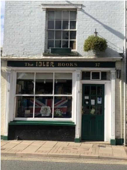
No 37 Grade II - Early Victorian wood shop front with traditional pilasters and fascia, traditional wood and glazed door to left of display window with wood doorcase and a tripartite transom fanlight over.
