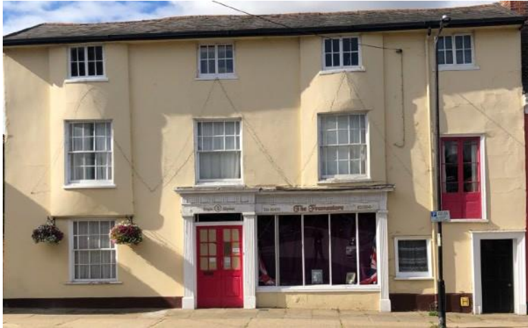
No 3 Grade II, Victorian. A later inserted shop window and door with a decorated Doric case with a triglyph frieze. Whilst not wholly sympathetic in its insertion into the building it is one of the more complete examples of a traditional shop window.
