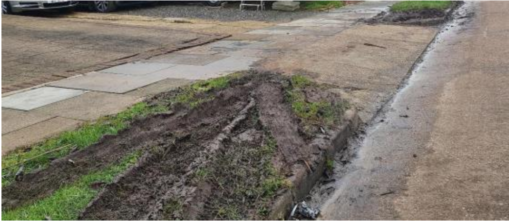
Example of damage to grass verges (source: Babergh and Mid Suffolk Parking Strategy 2022-2024)
