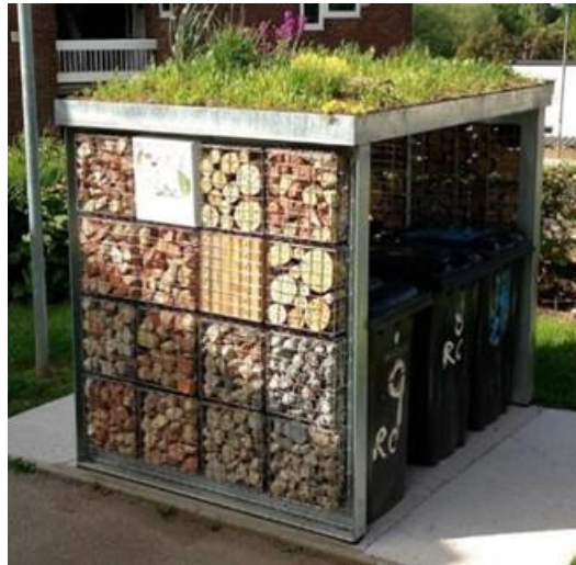
A bin store with green roof and habitat features (credit: Green Roof Shelters)
