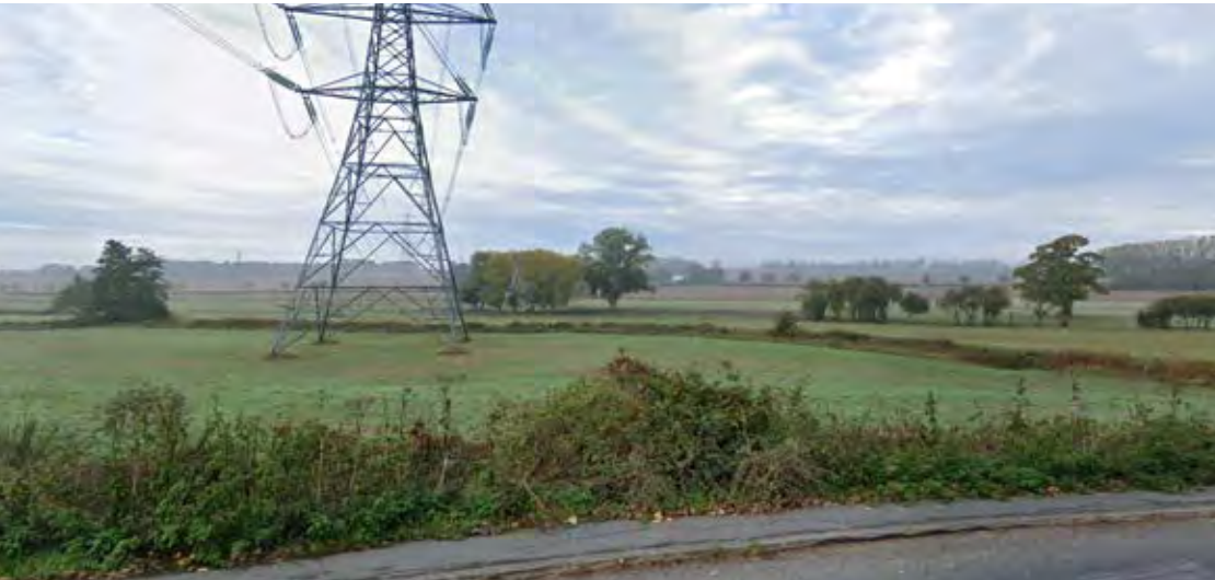
c Pylons are detracting features in an otherwise quintessential lowland river meadow scene.
