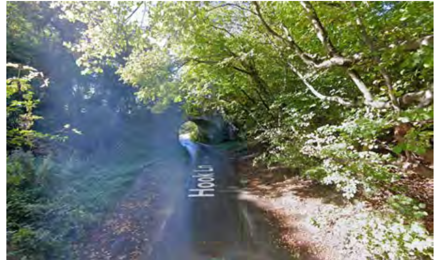
b Hook Lane as it passes beneath the old railway line
