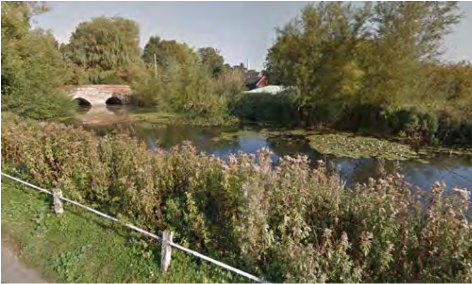
a Toppesfield Bridge is a scheduled monument and listed structure
