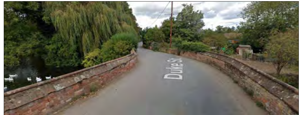
H- Toppesfield Bridge
