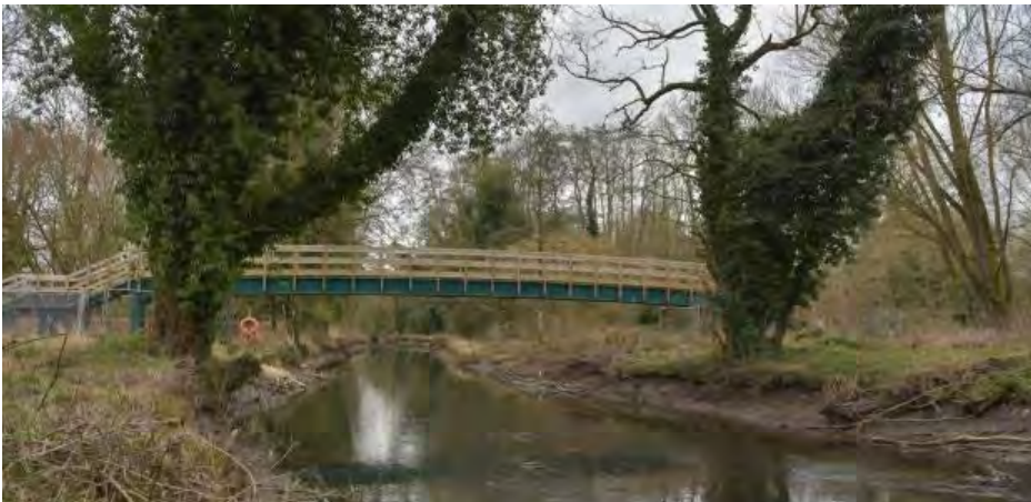
c The new footbridge linking the riverside walk with the heart of the town was provided through the McCarthy and Stone development on the adjacent site.
