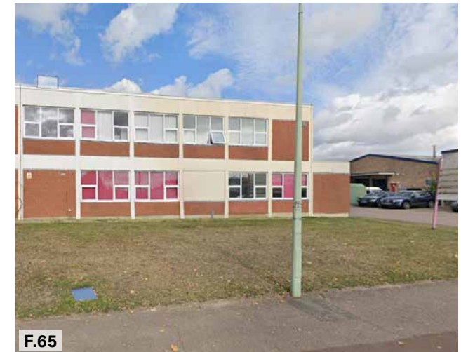
Figure 65: Typical red brick buildings.
