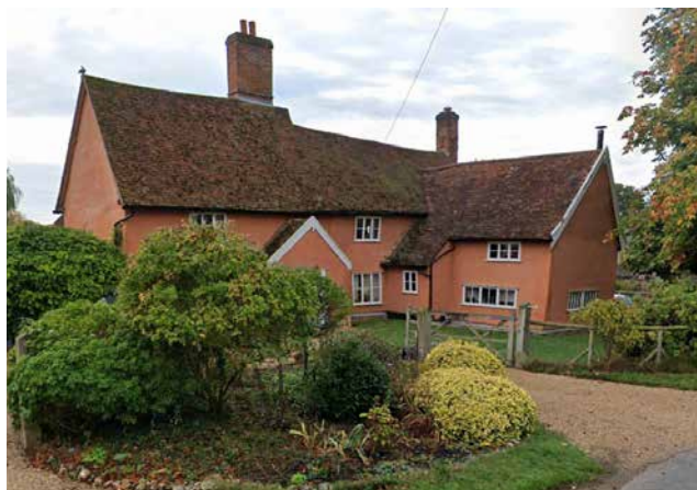
Figure 75: Historic property in Coram.
