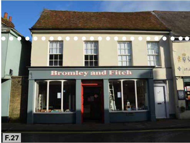
Figure 27: Example of two storey buildings on the High Street.
