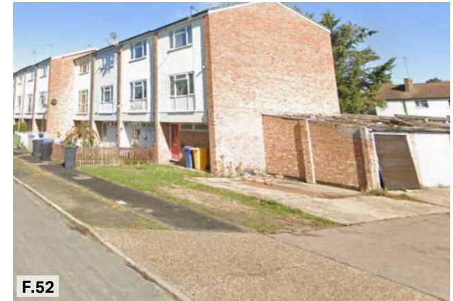
Figure 52: 3 storey 1970s terraces.
