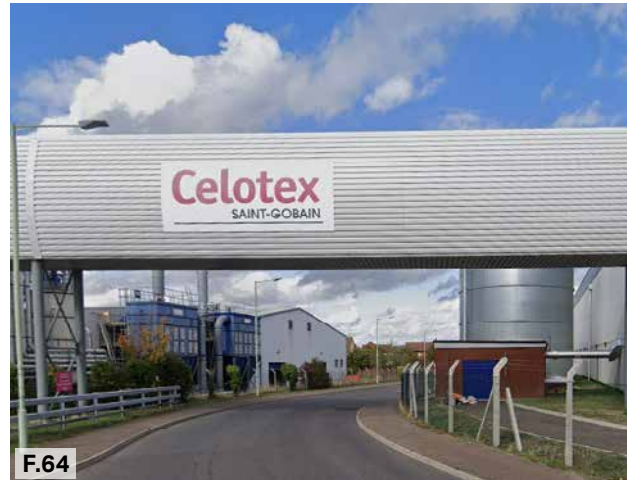
Figure 64: Overhanging building connecting two facilities.
