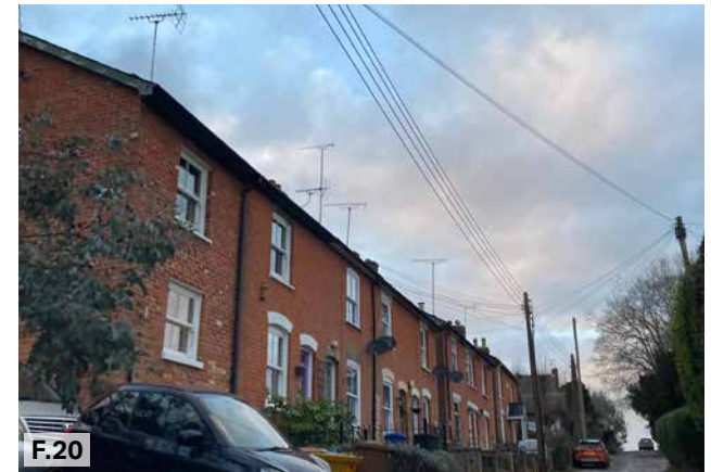
Figure 20: Terrace properties with a consistent roof line.
