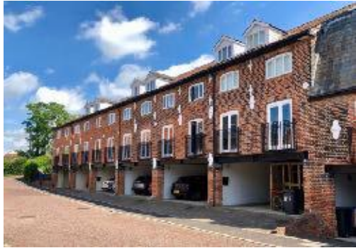
Converted Maltings in Station Yard
