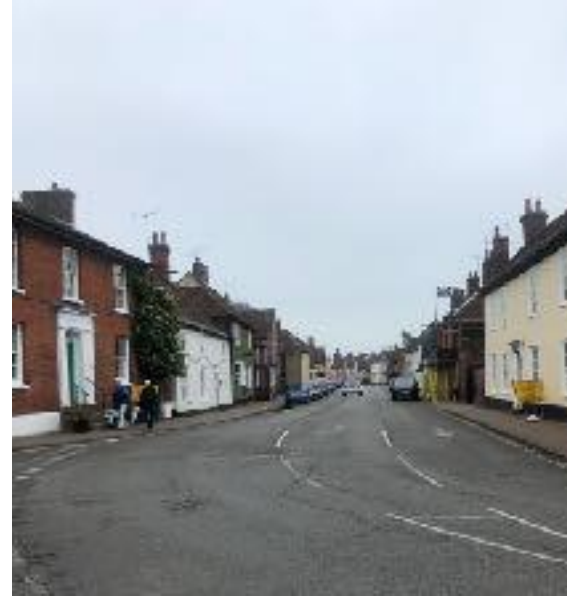
Entrance to town with dilapidated Bridge house & Grade II* C15 timber frame/paster houses View down the broad upper part of the High Street
