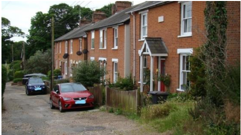
Castle Road; far south terraced housing
