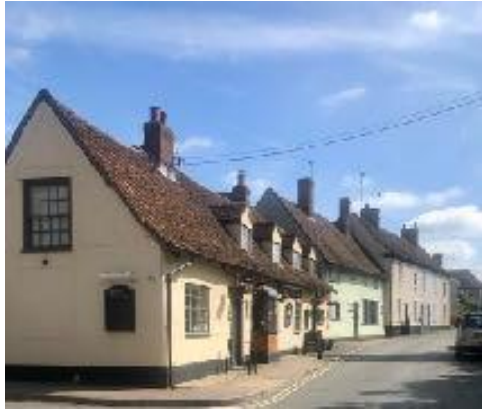
View eastward from Cock Inn
