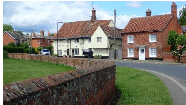
White Hart [Grade II*] & No 44 Bridge Street – [Grade II]
