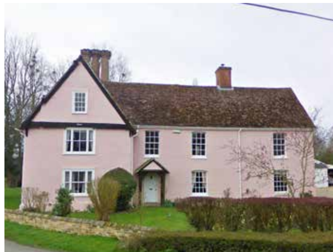
Figure 54: Building with a regular window arrangement.
