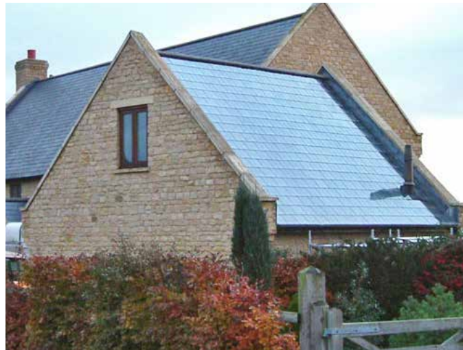
Figure 75: Retrofitted solar panels integrated sympathetically with a traditional building.
