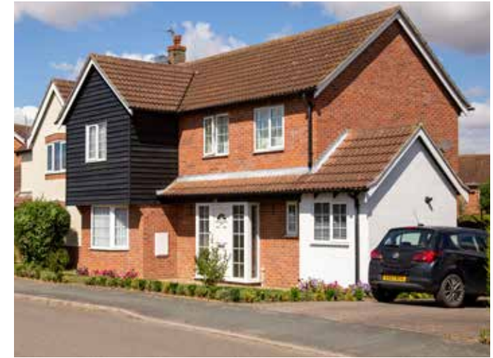
Figure 68: Single-storey side extension.
