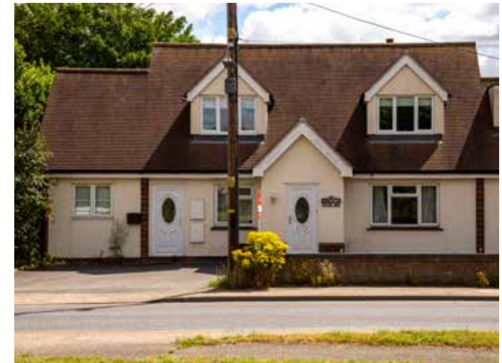
Figure 69: Single-storey side extension using the same materials as the original building.
