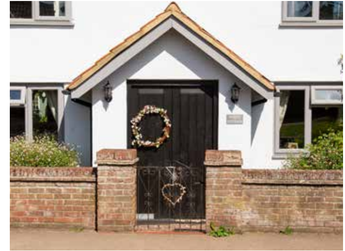
Figure 65: Wide, modern front door.
