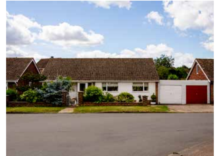
Figure 50: Bungalows with a simple form and pitched roofs.
