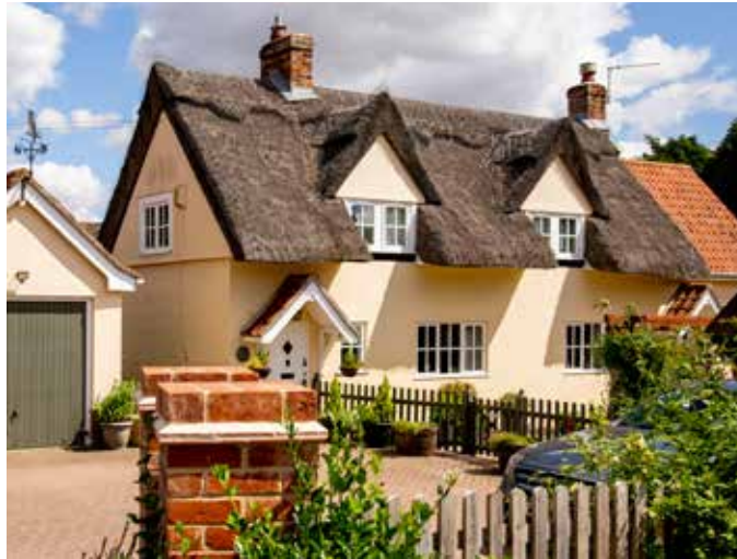
Figure 56: 2.5 Thatched cottage with dormer windows.
