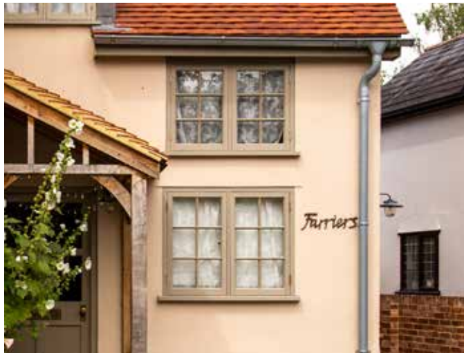
Figure 60: The same style of window used throughout the building.
