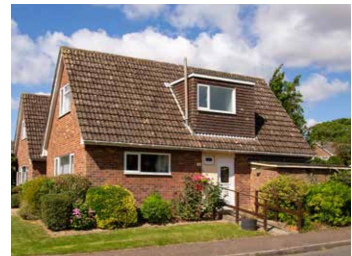
Figure 63: Out of scale dormer window with a flat roof should be avoided.
