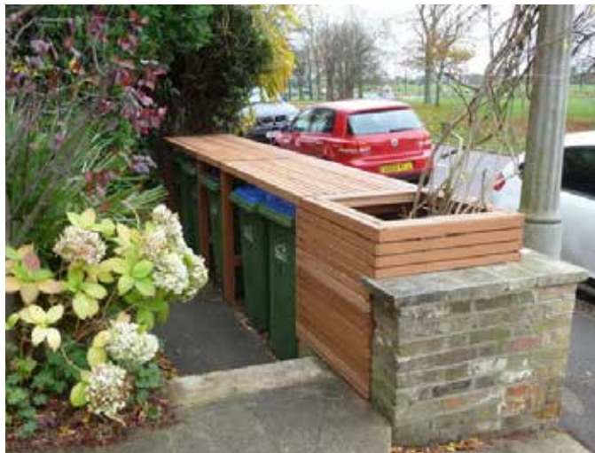
Figure 83: Waste bin storage used as a boundary treatment.
