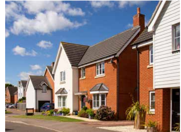
Figure 57: Recent development using a variety of materials such as red brick, white render and white weatherboarding.
