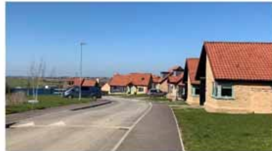
Community Land Trust housing in Cambridgeshire
