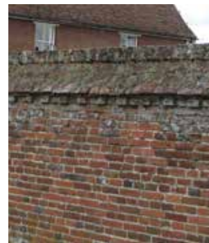
Red brick wall with saddleback brick coping
