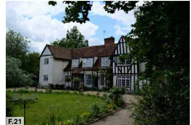
Figure 21: A two-storey dwelling with an off-white façade, black half-timbering and a pantile roof.
