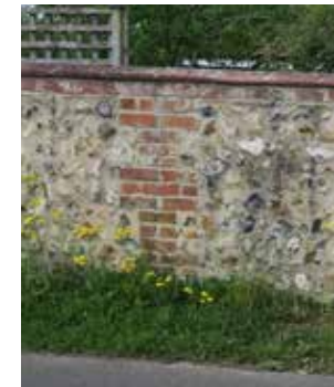
Red brick wall with flint infilling
