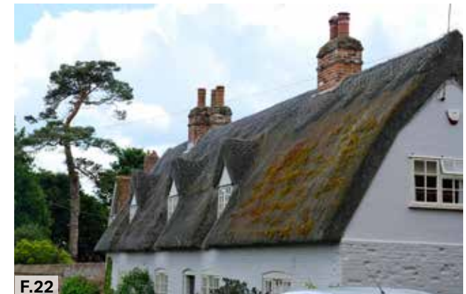
Figure 22: One-storey dwelling with a thatched roof and white-rendered facade.
