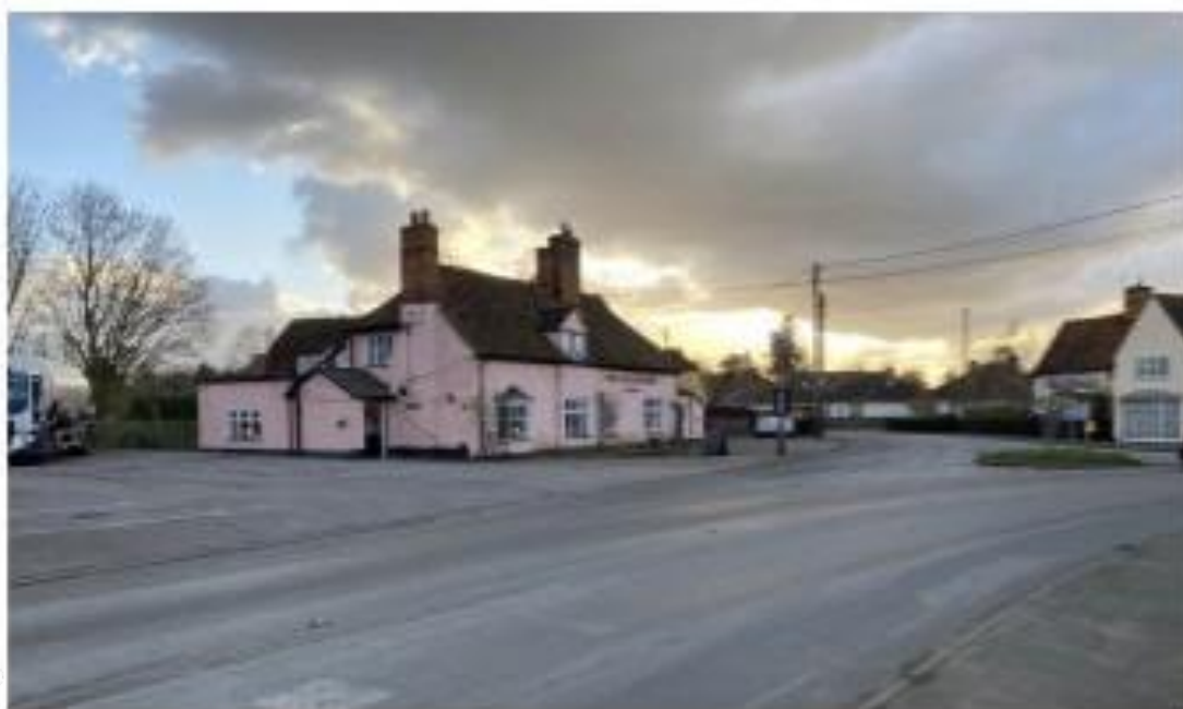
Figure 243: The car parking and setting of the Carriers Arms and junction between Gaston End and Gaston Street,
