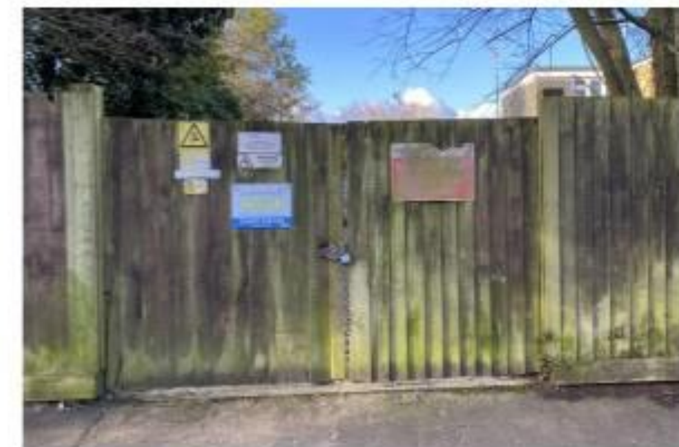
Figure 245: Unremarkable utilities fencing close to the Box Iron.
