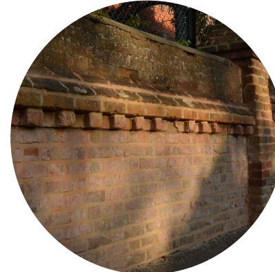
RED BRICK BOUNDARY WALL
