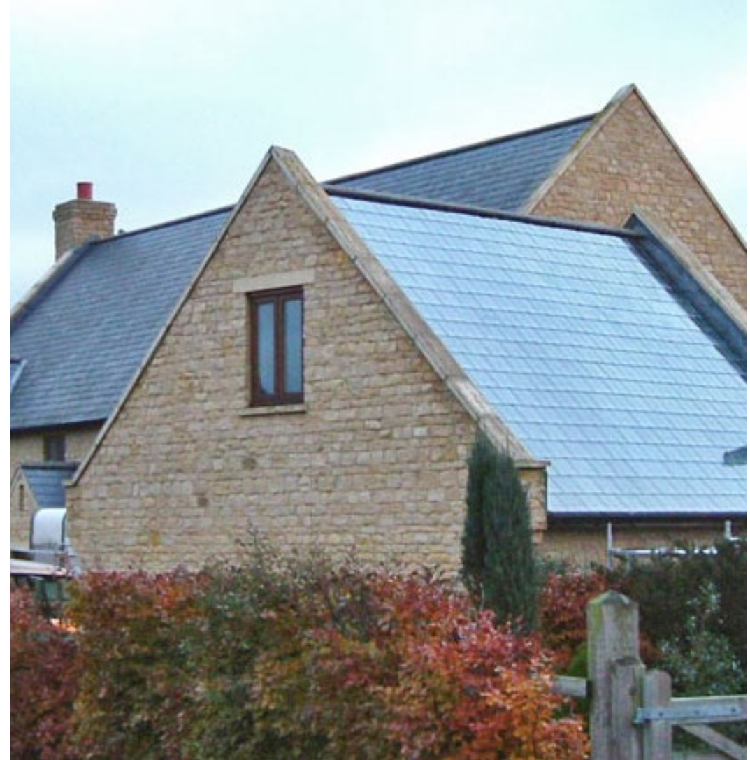
Figure 42: Solar panels do not need to be obtrusive. Here, they make a positive contribution to appearance by blending with roof tiles.
