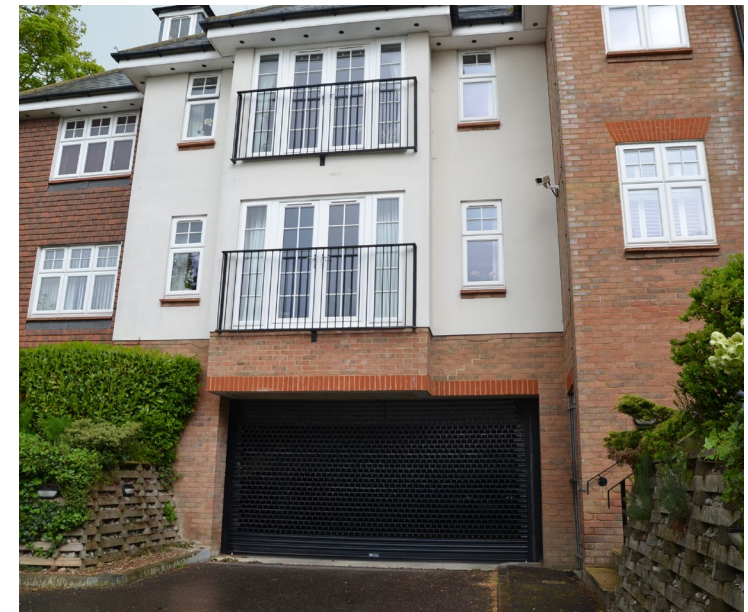
Figure 55: Apartment building with undercroft parking entrance partly screened with landscaping.
