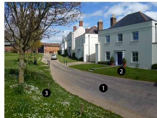
Figure 50: Examples of edge lanes in Dorchester, with low-speed roads shared between motor vehicles and cyclists, and opportunities for on-street parking (note: some localities may prefer clearly defined footways and parking bays).
