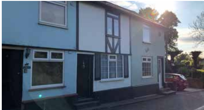
Example of terraced housing in Copdock village
