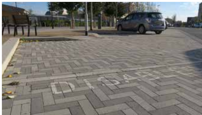
Disabled parking bay in Cambridge with ramp for easy wheelchair access.
