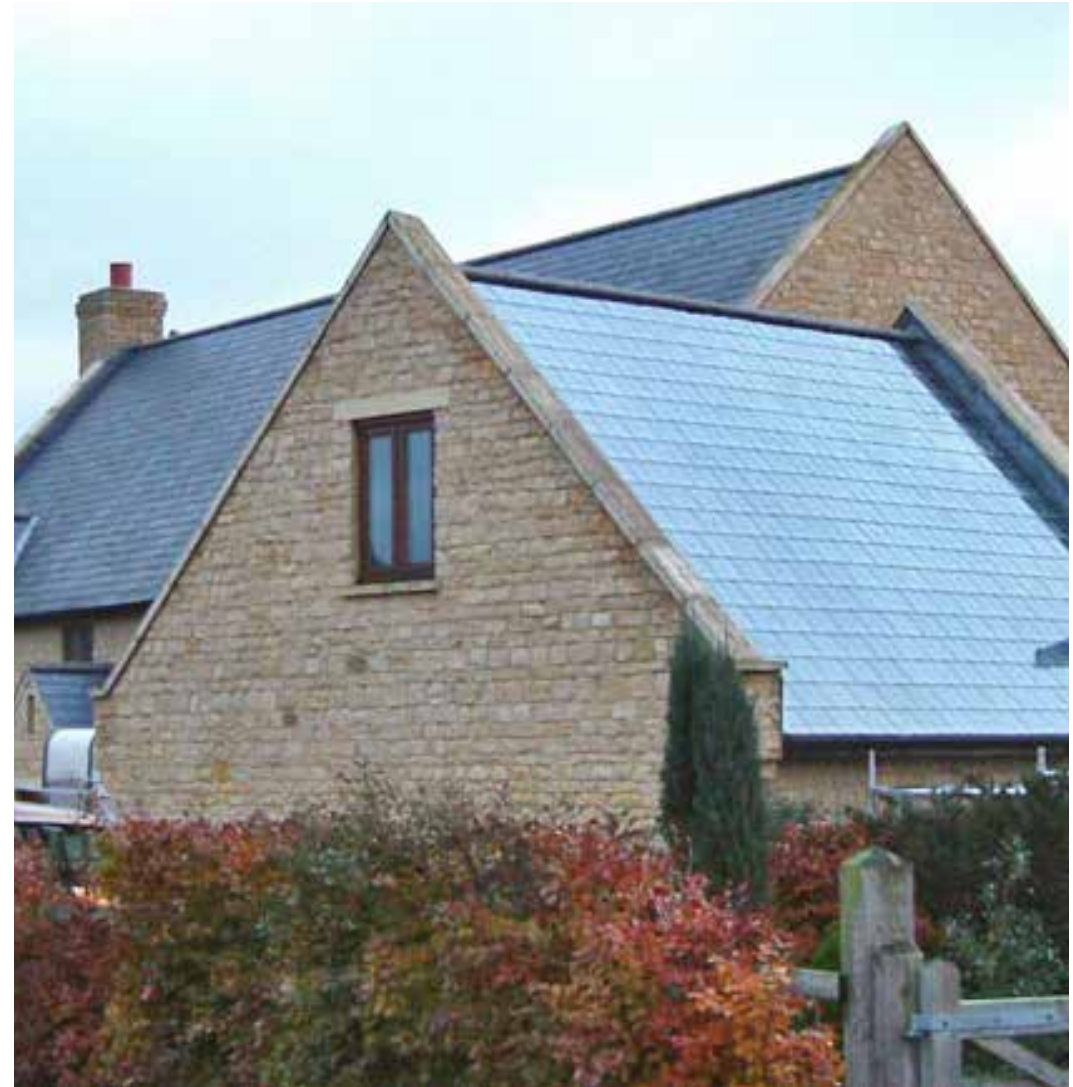
Solar panels do not need to be obtrusive. Here, they make a positive contribution to appearance by blending with roof tiles.
