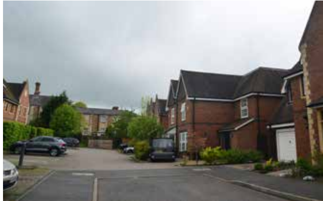
Contemporary development with a mix of courtyard parking (centre) and garages (right).
