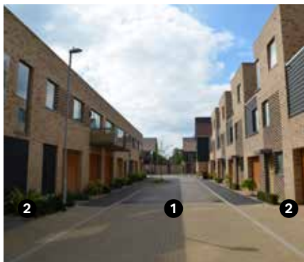
Example of a lane/ private drive in Cambridge, with a shared surface for all road users.
