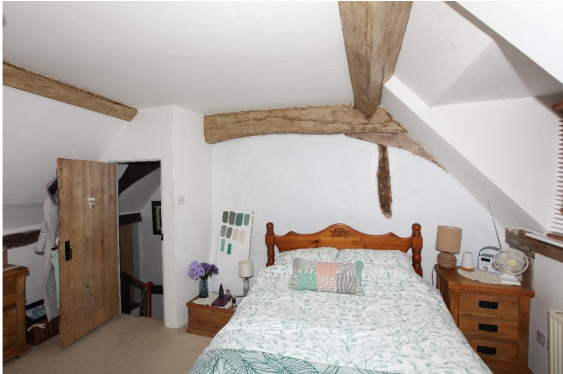
Illustration 4. The chamber over the hall showing the A-frame roof truss against the high-end chimney. The pegged collar braces are original but the clasped-purlins are hidden by later pine boards and the light colouring is modern. A-frames of this kind were designed to avoid the need for inconveniently low tie-beams spanning the roof-plates which are visible to left and right and lack dovetails for tie-beams above the posts.
