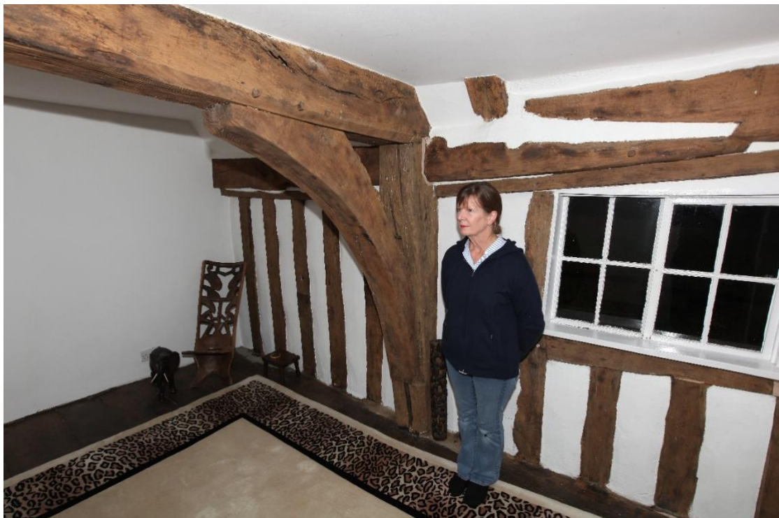
Illustration 25. The eastern arcade-plate contains a long splayed scarf joint of standard 14 th century form. The heavy, unchamfered arched brace and tie-beam appear to be original features but the post was replaced when the present wall was built.
