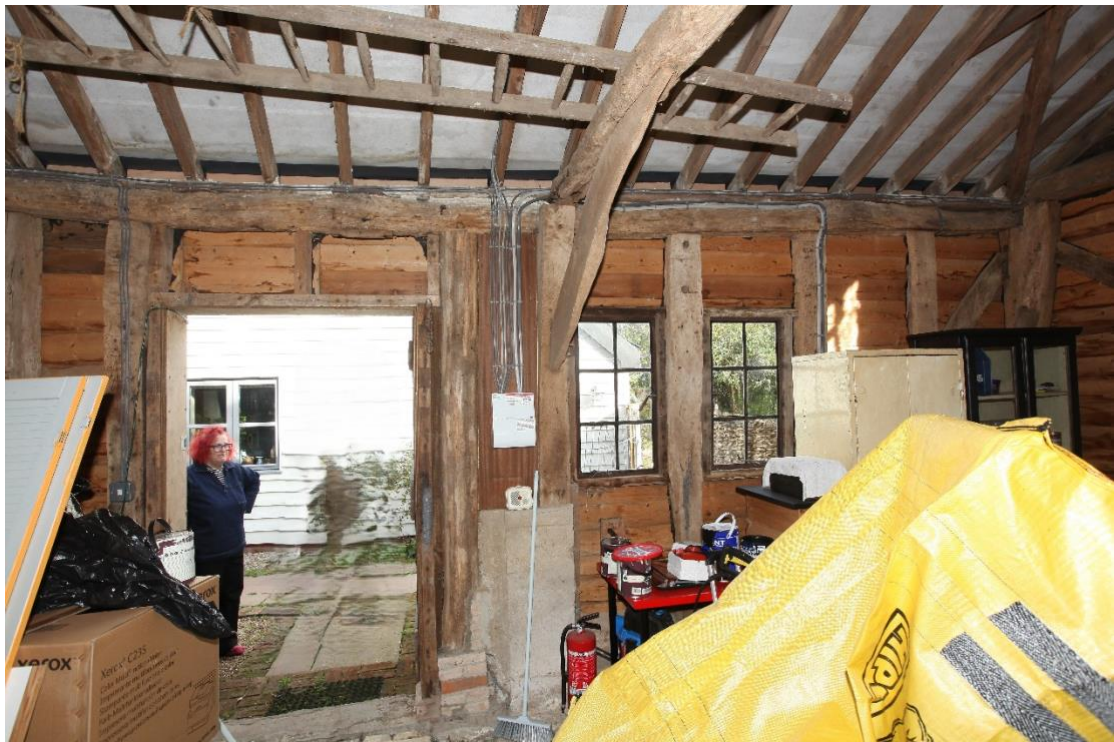
Illustration 5. The northern interior of the small three-bay 16 th century threshing barn showing an intact arch-brace with externally trenched corner braces on the right. This unusually small structure is contemporary or broadly contemporary with the house.
