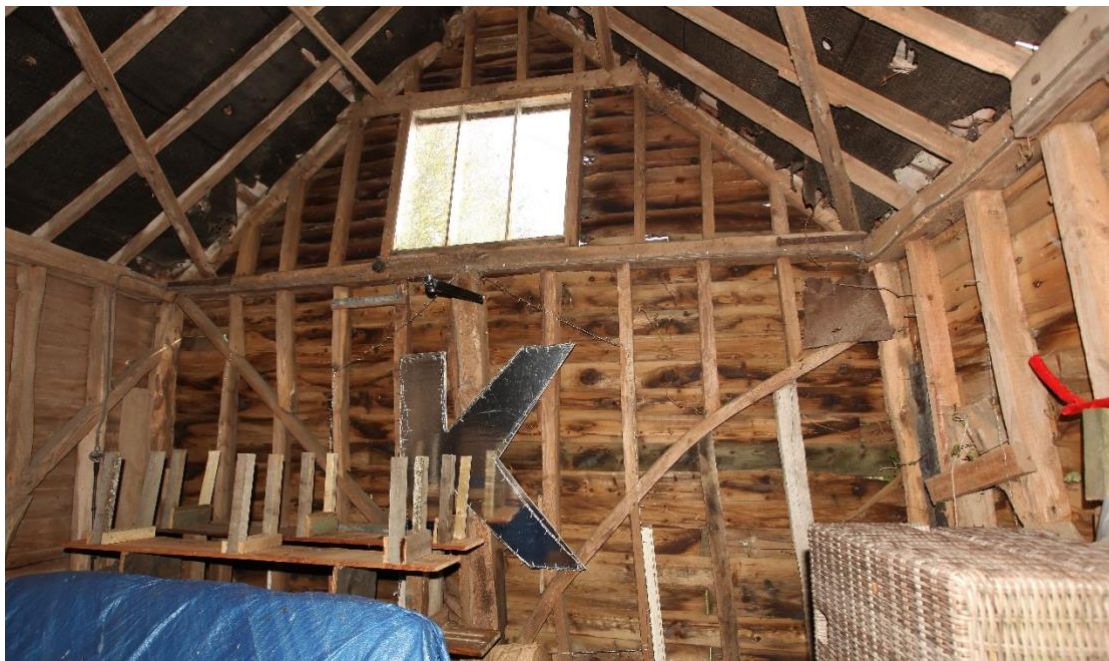
Illustration 7. The intact mid-19 th century framing of the barn's eastern internal gable.
