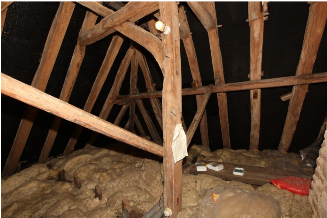
Illus. 35. The crown-post on the tie-beam between the two bays of the hall, as seen from the rear (north). The right-hand brace has been lost and the lower struts and purlins are insertions (although the original rafters are in excellent condition).
