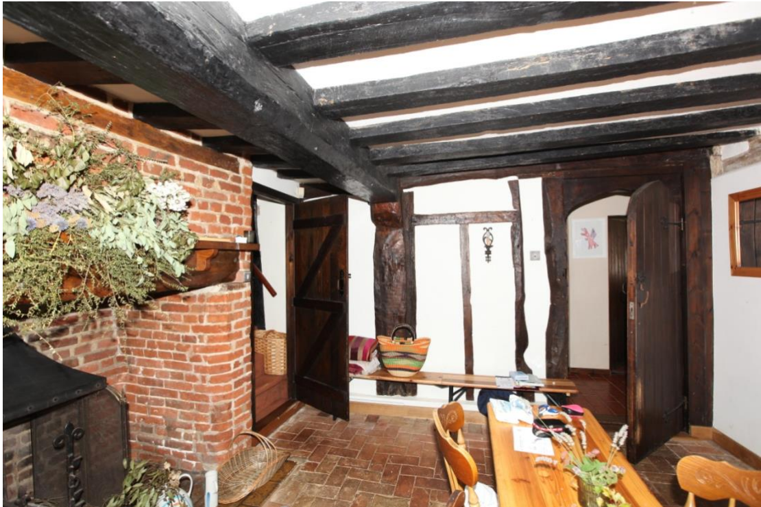
Illus. 34. The rear wall of the hall to the right of the inserted chimney with the original arched head of the back door to the cross-passage on the right. Its jamb preserves the double-pegged sill mortice of a large window to its left where the timbers of an inserted additional door can now be seen. The high-end bay to the left of the storey post is almost filled by the later chimney.
