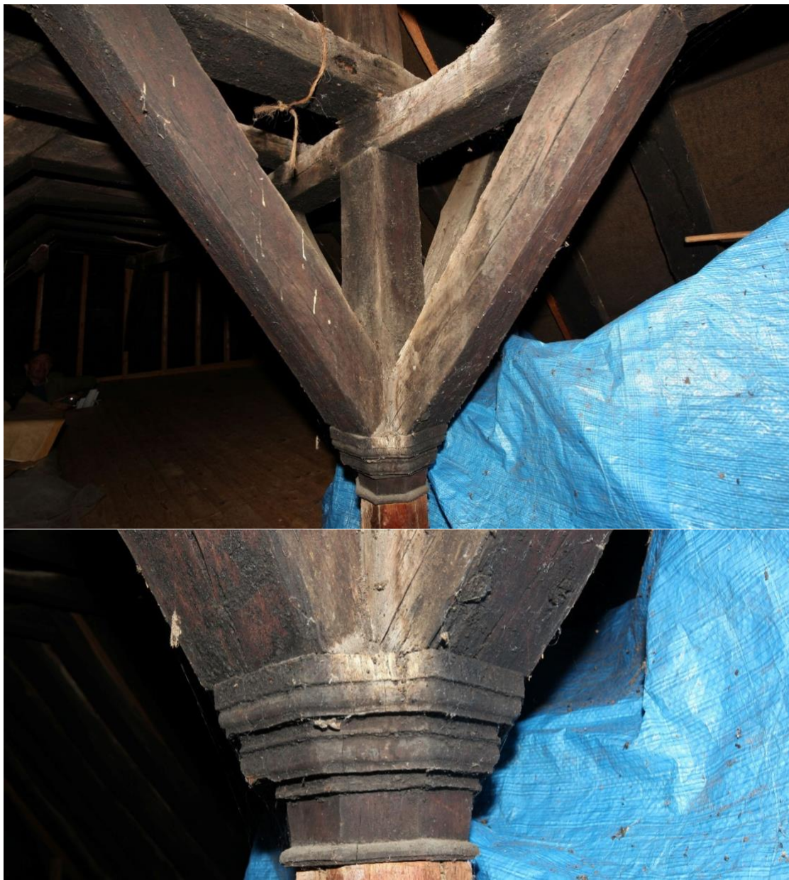
Illustration 23. The fine central crown-post of the aisled hall with a detail below.
