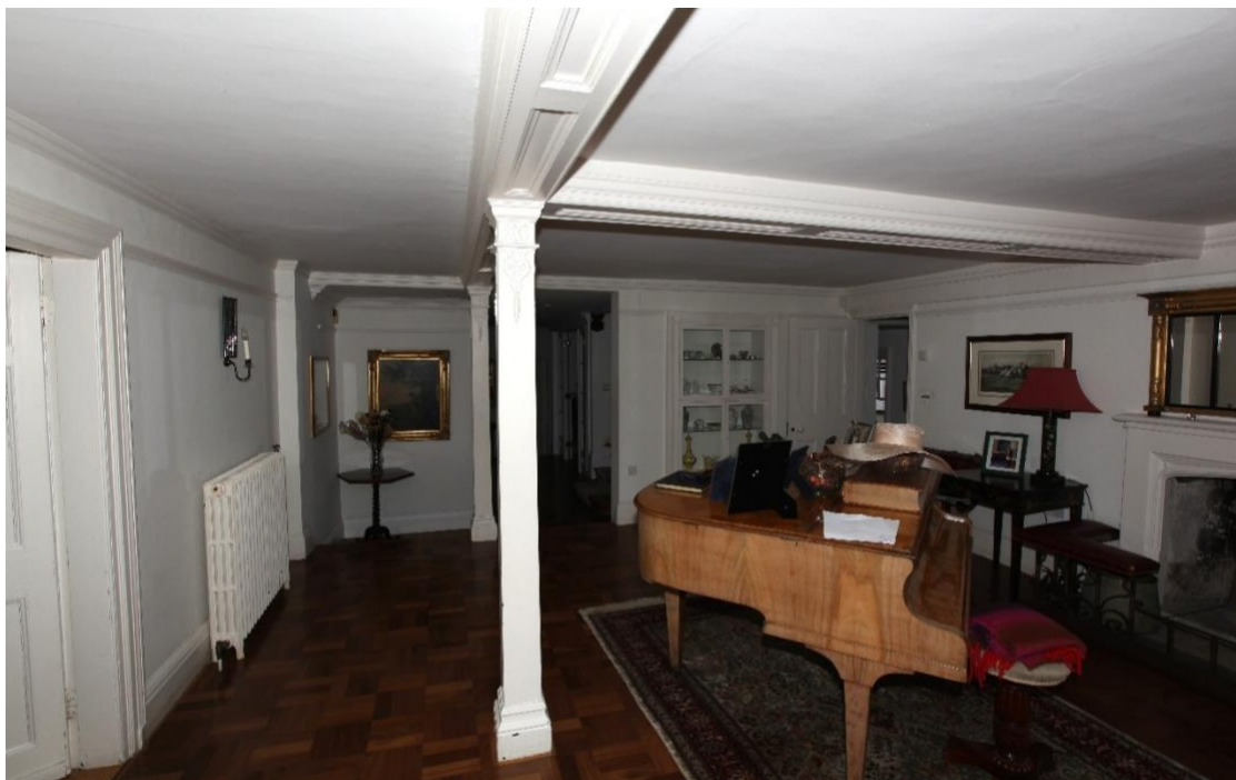
Illustration 15. The central entrance hall of Bentley Park with the southern parlour to the left. The panelling of the principal ceiling joists is convincingly Georgian rather than late-Victorian and suggests the present porch opens into a former cross-passage with a high-end chimney on the right. No early framing is exposed in this part of the house, but there is evidence of an original axial partition in the visible 16 th or early-17 th century framing of the kitchen beyond the chimney which indicates it was designed as a pair of service rooms – in which case the chimney may occupy the original cross-passage of a house that subsequently exchanged the functions of its end-bays in a manner often seen elsewhere.
