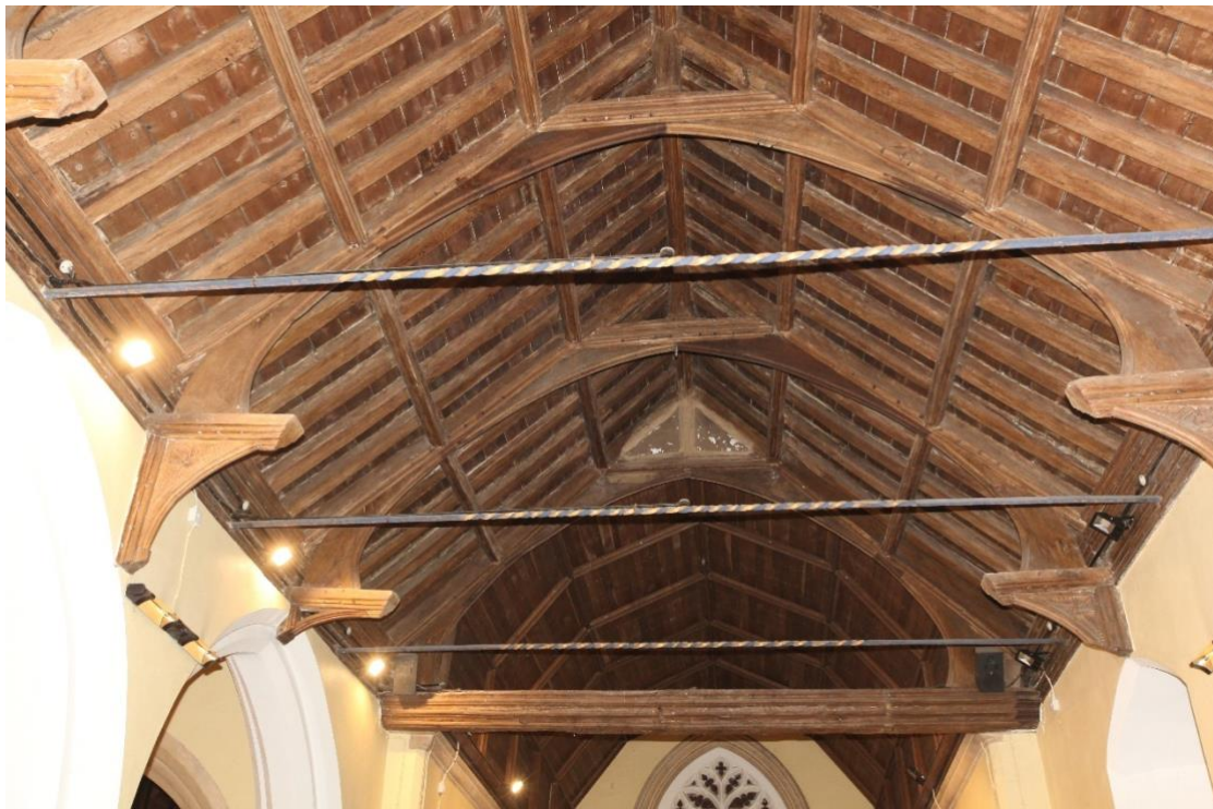
Illustration 12. The fine 15 th century false-hammerbeam roof in the nave.
