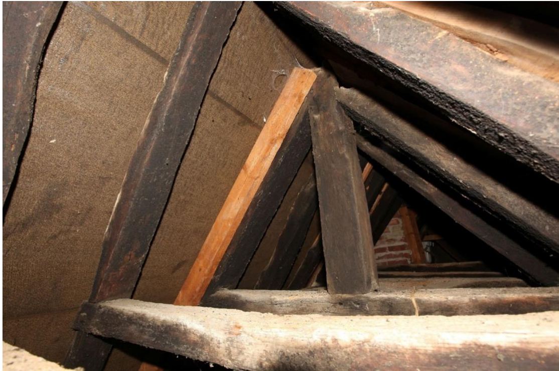
Illustration 24. A single post above the crown-post's collar would have projected above the ridge to support a louvre that was probably largely decorative but also served as a smoke vent. The timber is double pegged to the collar and pegged mortices secure the rafters on both sides.
