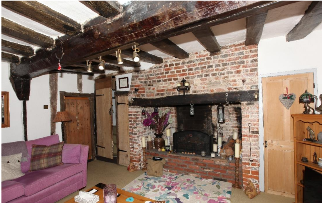
Illustration 2. The two-bay central hall of Potash Farm showing its substantial binding joist with step-stopped chamfers and plain common joists. The 'inglenook' cooking fireplace backs onto the parlour bay which was not inspected. Unusually heavy framing of this kind is typical of Bentley and probably reflects the fact that most of its early houses belonged to the Tollemache family and were built using timber from the parish's extensive ancient woodland.
