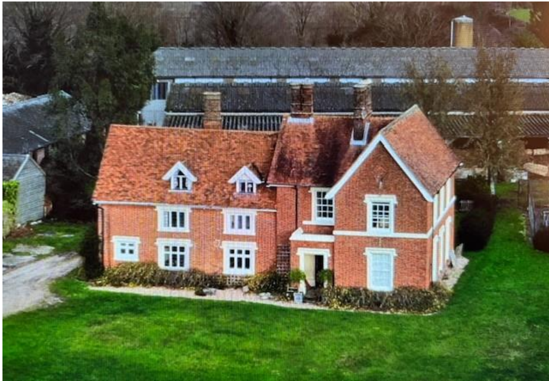
Illustration 27. The high-quality Victorian Mock Tudor exterior of Falstaff Manor in a supplied aerial image taken from the south. The polygonal chimneys, hood mouldings and Flemish Bond brickwork appear to be contemporary with the eastern wing on the right but were added to an older and lower timber-framed range on the left.
