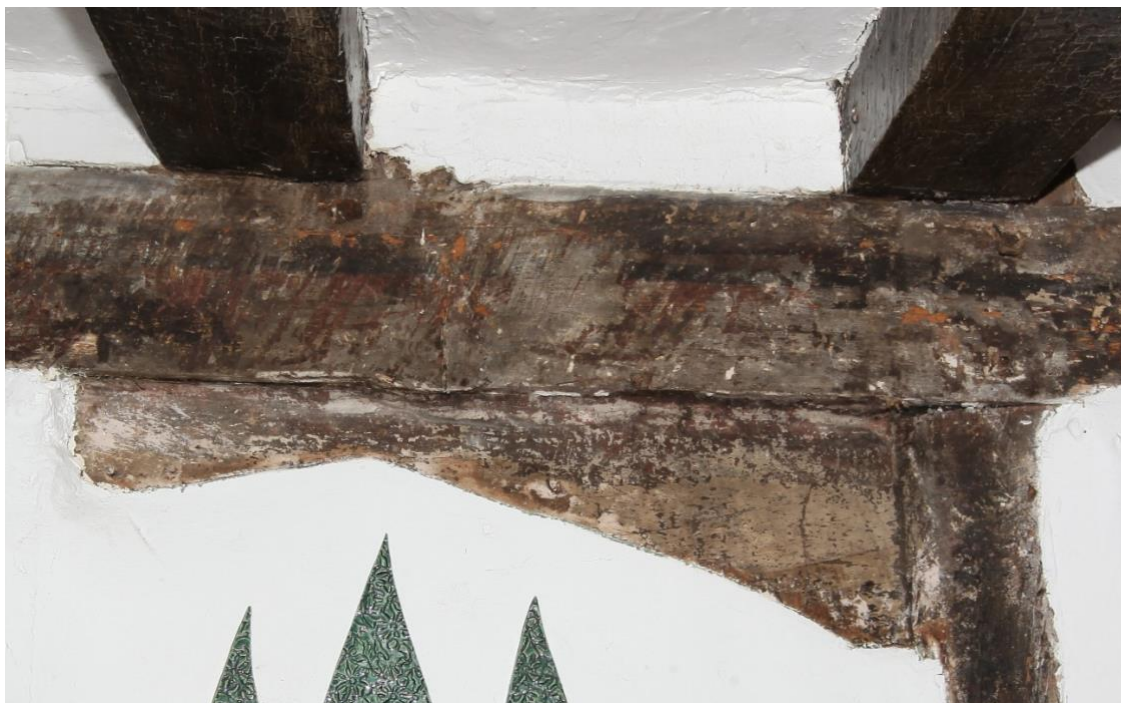
Illustration 3. A detail of the original arched service door in the southern wall of the hall showing horizontal black lines and a red background on the mid-rail above. Other designs lie beneath and could be revealed by professional cleaning. These rare and historically significant wall paintings may be contemporary with the mid-16 th century house and are certainly no later than the early-17 th century.
