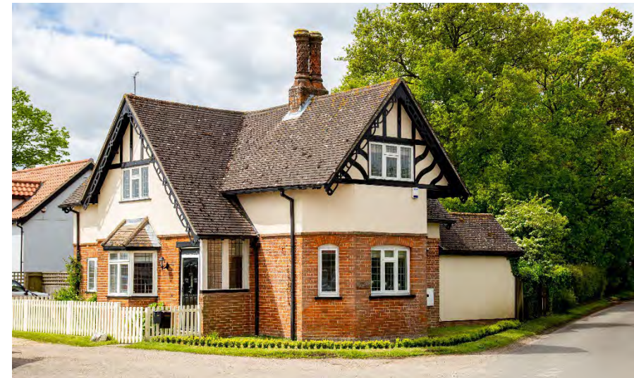
Octagonal chimney shafts and gables with bargeboards contribute to character.
