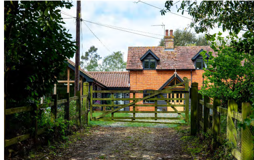
Modern extension of The Gardens on Bury Road.
