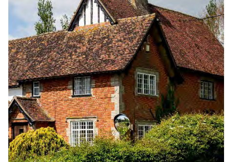
Red brick with white brick corner detailing
