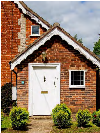
Timber door with simple doorcase
