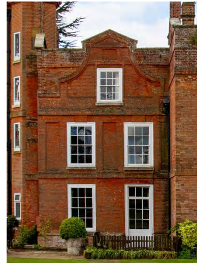
Sash windows with glazing bars
