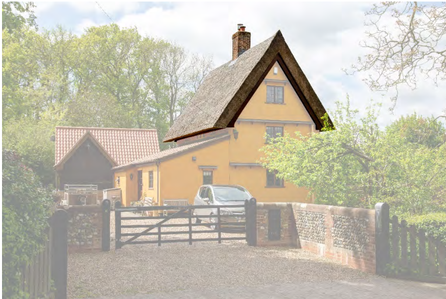
Brewers Cottage, an example of a steep pitched thatched roof with a central ridge and square chimney stack.
