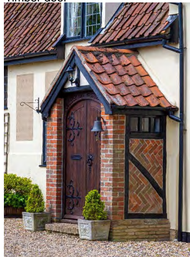
Timber doors with timber frame and brick porch
