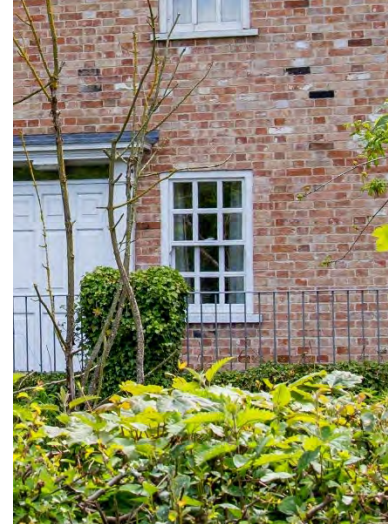
Sash window with glazing bars
