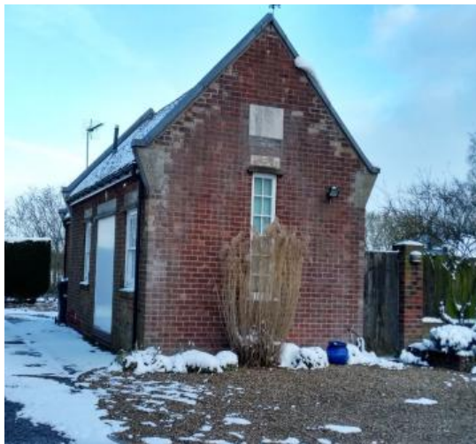
c) The Village Pump House
