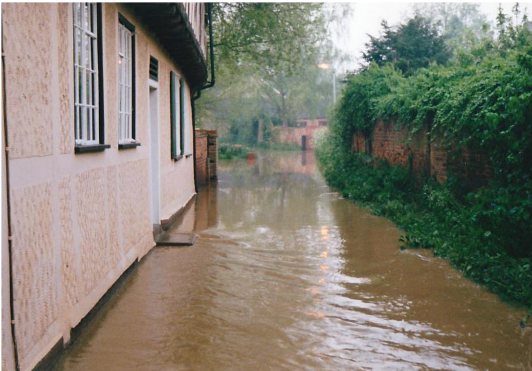
May 2000 floods – see above and below (Butcher’s Lane and the Causeway).
