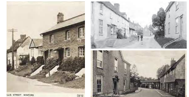
Variation in built form and enclosure as settlement evolved over the years at Boxford
