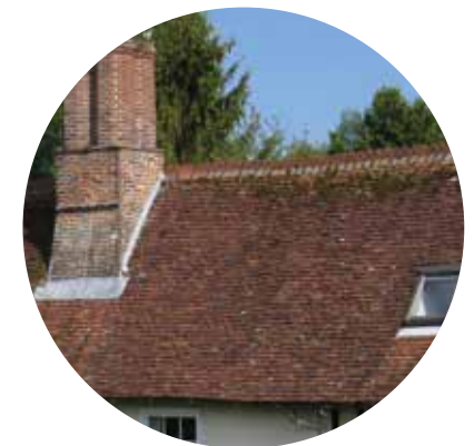
CLAY RED FLAT TILED ROOF WITH RED BRICK CHIMNEYS
