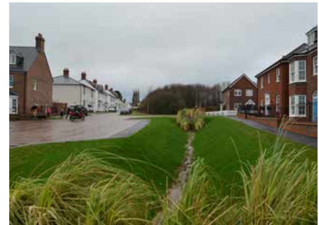
Figure 74: Example of SuDS designed as a public amenity and fully integrated into the design of the public realm, UK.
