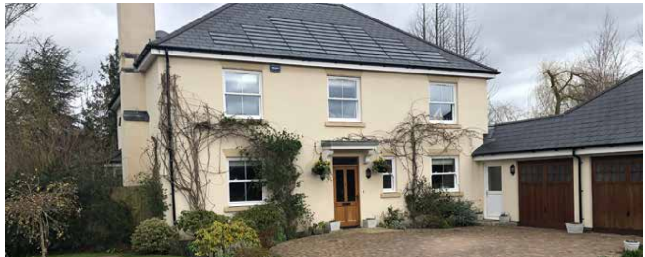
Figure 76: Use of shingle-like solar panels on a slate roof, with the design and colour of the solar panels matching those of the adjacent slate tiles in Lingfield, Surrey.
