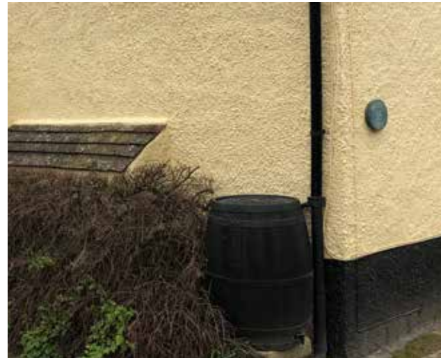
Figure 83: Examples of water butts used for rainwater harvesting in Reach, Cambridgeshire.
