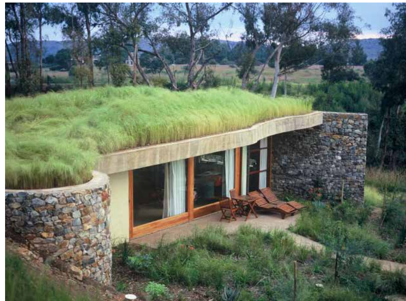
Figure 82: Green roof integrating the building with the countryside.
