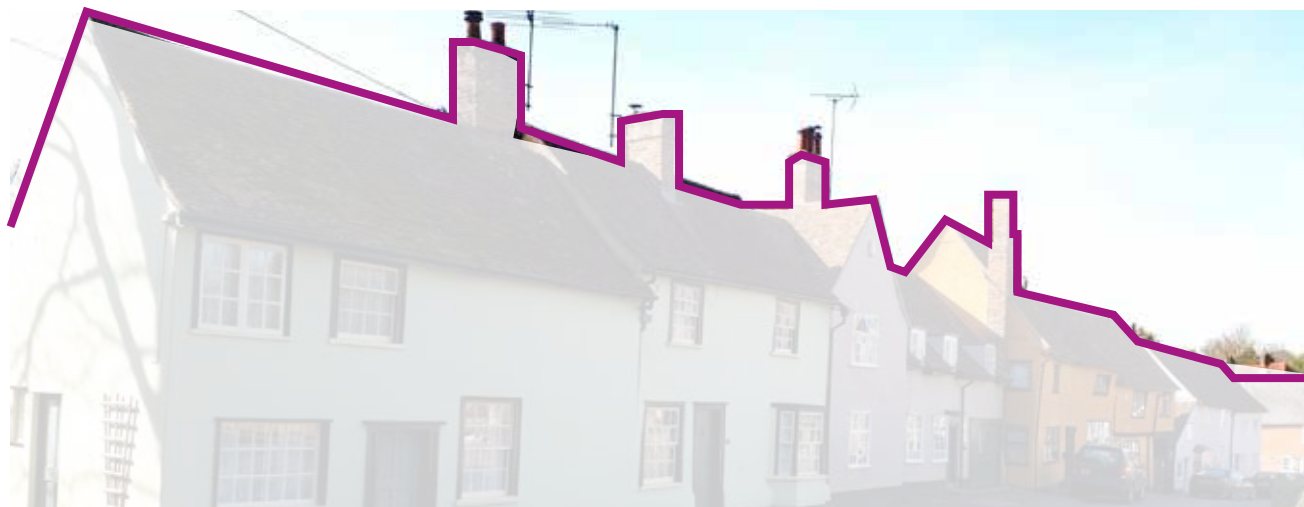
Figure 62: Within the historic core, the roofline is continuous, due to the building groupings, creating an interesting visual result.
