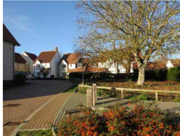
Figure 14: Use of different colours in materials on the public realm, as well as appropriate signage to indicate the footpath entrance, improve legibility and encourage people walking and cycling.
