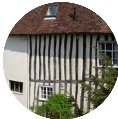
TIMBER-FRAMING WITH WHITE RENDER INFILLS
