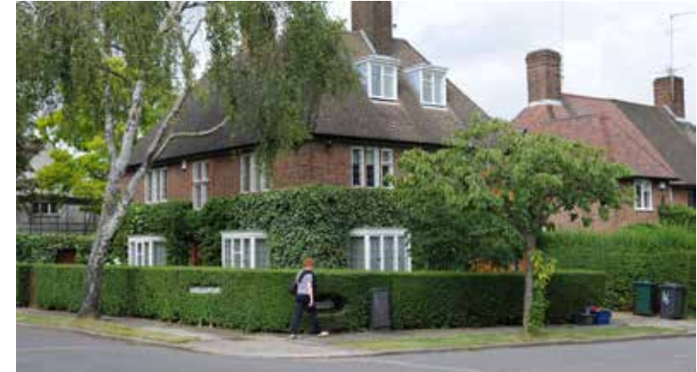
Figure 58: Example of a corner addressed by a detached house with windows on both streets to enhance natural surveillance and physical boundary treatment to add a level of privacy as well.
