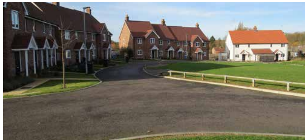
Figure 61: Green open spaces surrounded by buildings can create an enclosed environment reflecting the character of Boxford village.
