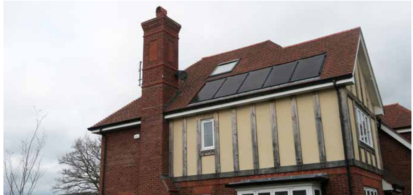
Figure 75: Integration of solar panels on the south-facing pane of the roof of a new house in Lingfield, Surrey.
