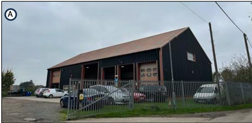
figure 101: Capel Station Garage is of no historic or architectural interest and located at an important entry point to the area (where the Victorian Capel railway station was once located). Note also unattractive palisade fencing.
