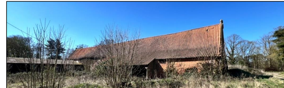
figure 136: Bentley Hall Barn [Grade I listed building]
