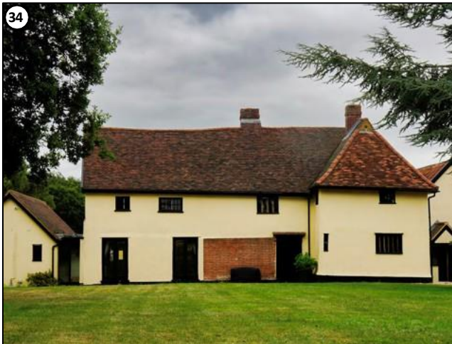
figure 46: View of the grade II* listed Bentley Old Hall.
