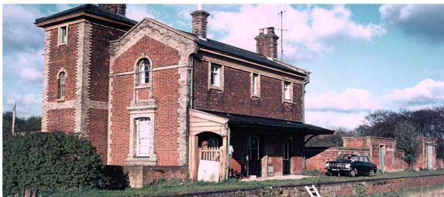
Figure 21: Photograph showing Capel Station's western and northern elevations
