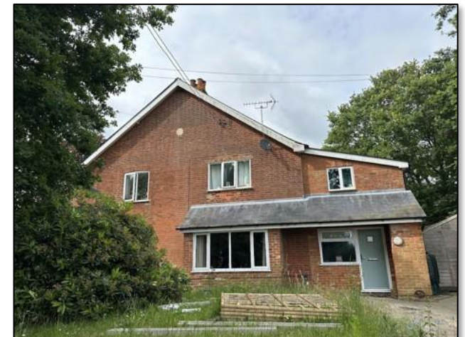
figure 112: Inappropriate plastic windows and altered fenestration to 5 Falstaff Cottage
