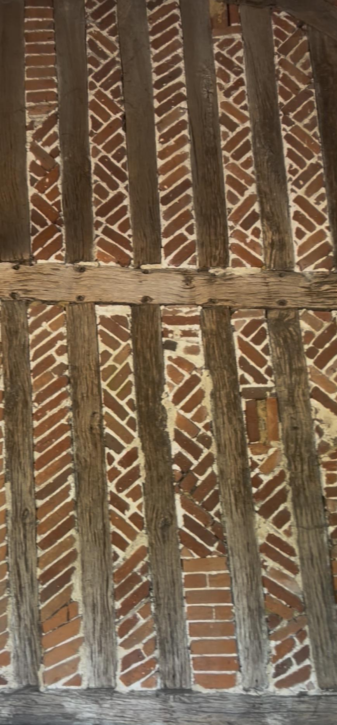
timber frame with brick noggin Bentley Hall Barn
