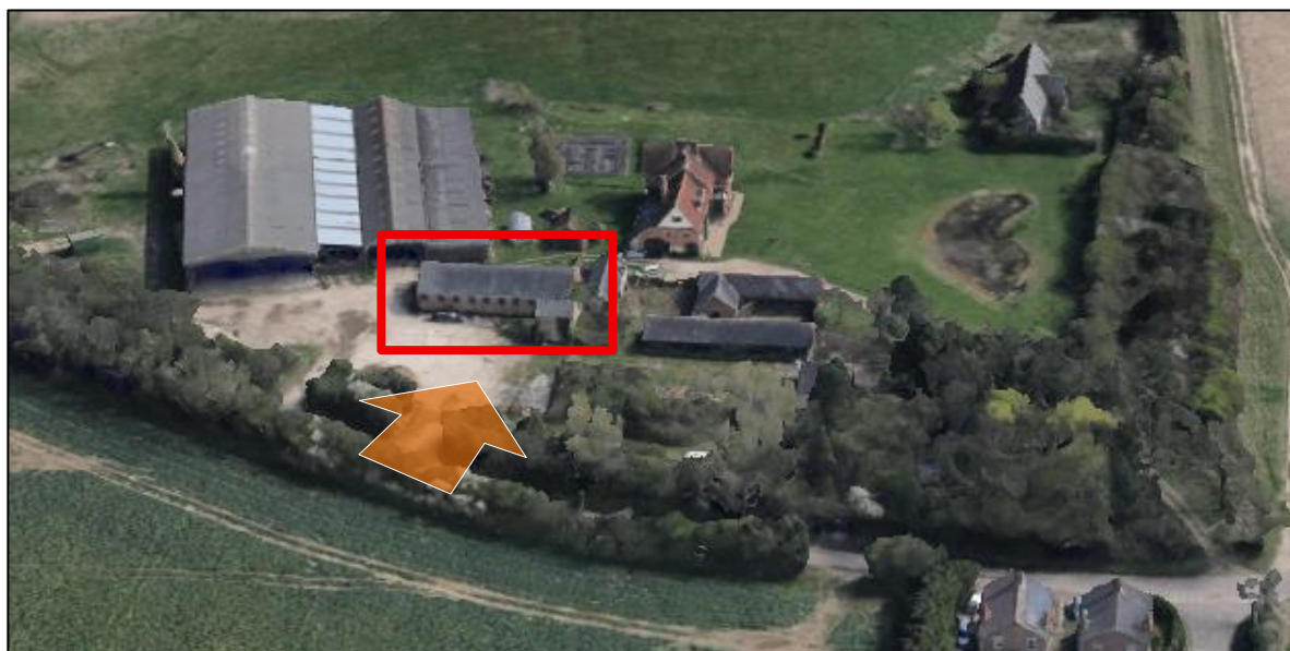
figures 181: Brick farm buildings rear of Falstaff Manor non-designated heritage assets
