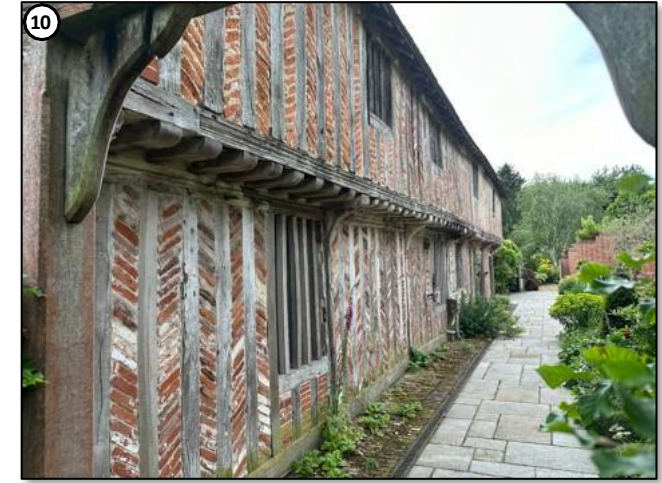
figure 39: Bentley Hall Stables/Meeting Hall showing herringbone-brickwork and closely spaced joists.
