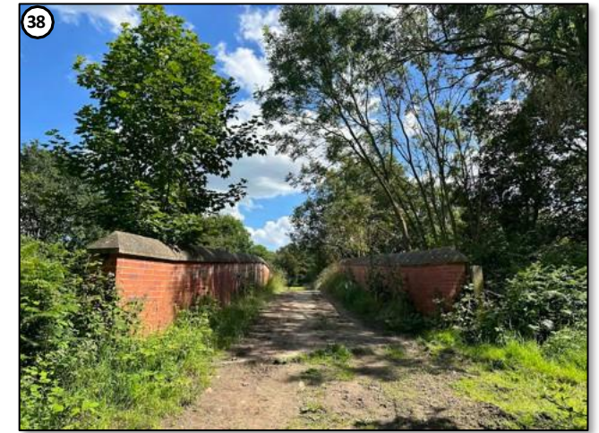
figure 48: Railway bridge with earlier fabric at track level.
