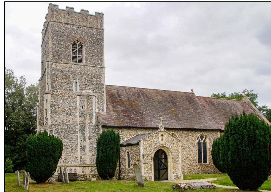
figures 190: St Mary's Church Grade II* Listed Building
