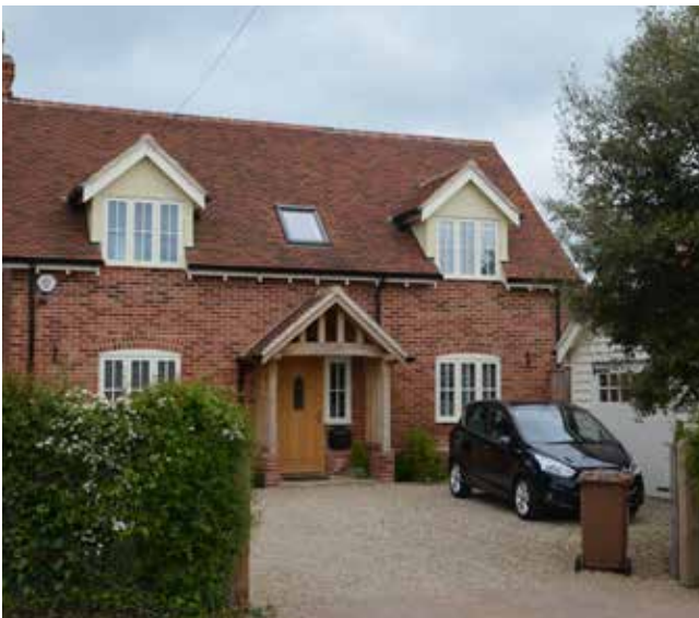
Figure 20: Detached house on the Street
