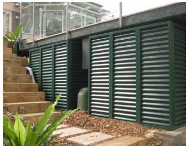
Figure 46: Examples of concealed tanks used for rainwater harvesting
