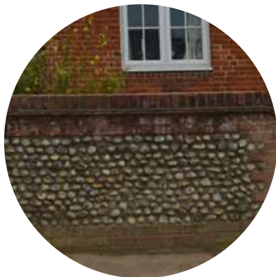
FLINT WALL WITH RED BRICK CAP
