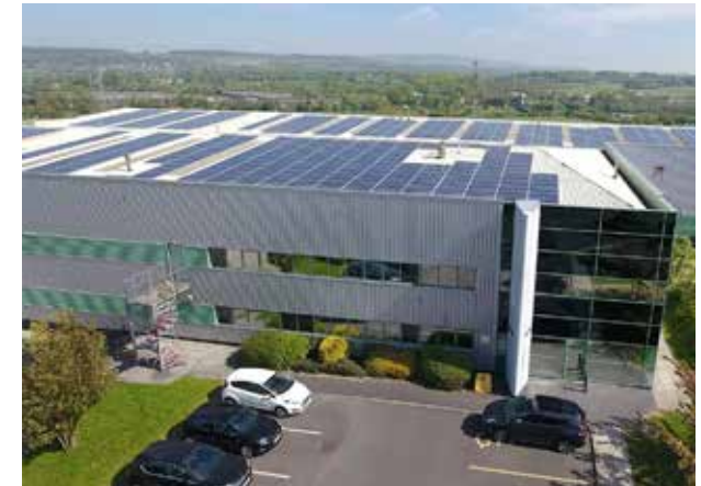
Positive example of large industrial building with integrated solar panels on the roof
