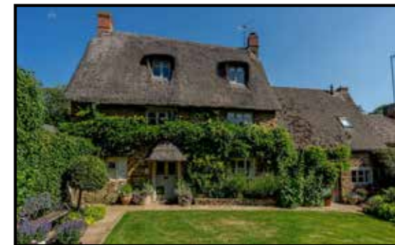
Green roofs and walls should minimise power use and do not need to be heavily engineered solutions. Climbing plant species such as vines are a traditional way of achieving the same effects
