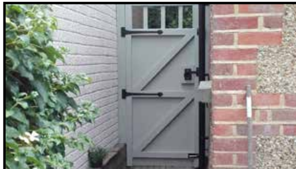
Access gate to back gardens, that provides a clear route for refuse bins to be moved from back gardens to the front of the property for collection
