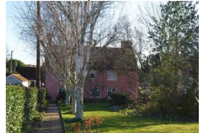
Illustrative diagram and example in the village of housing with large front gardens.
