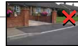
Interrupted pavements over driveways
