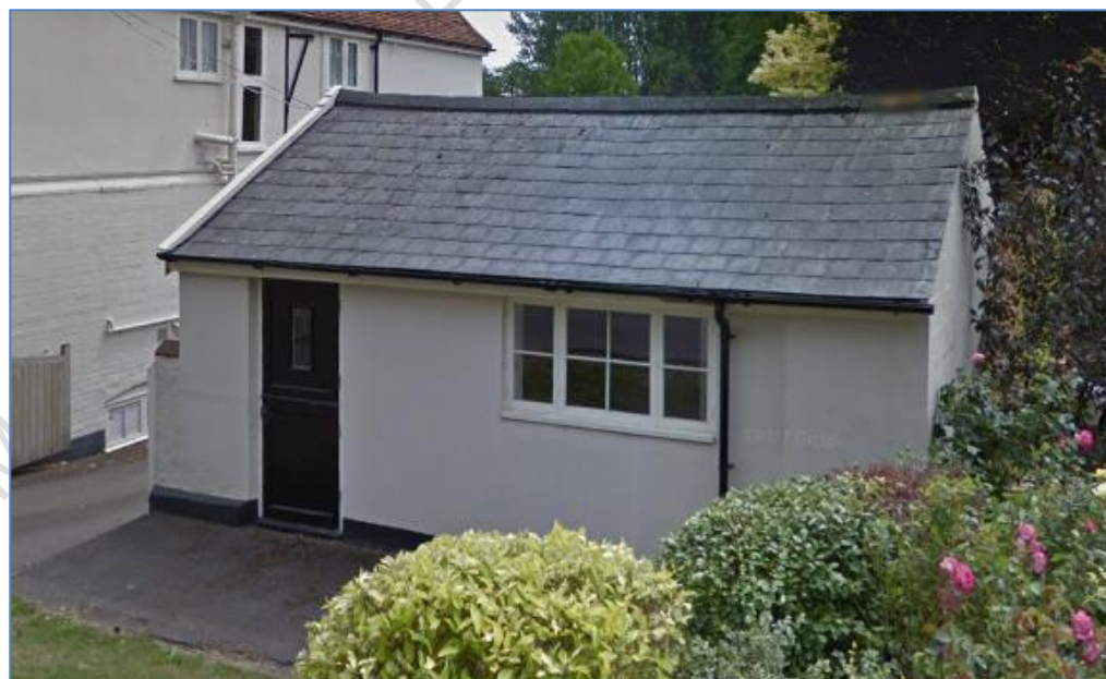
Small outbuilding utilising natural blue/grey slates on its roof and a black clay ridge tile. Blue/grey slates are traditionally sourced from Wales.
