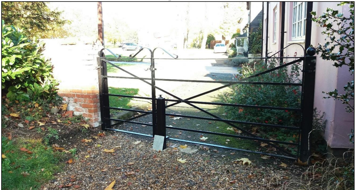
Metal five-bar gate; elegant and discreet in appearance. Most likely to be seen on a formal drive to a 19 th century residence. Used successfully, in this instance, in combination with a historic red brick boundary wall.
