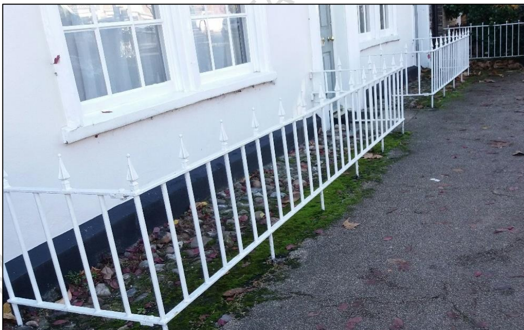
Metal railings are formal in character and are more often associated with 19 th century buildings, in historic towns, or surrounding parkland or estates. They provide a balanced treatment, marking the boundary but allowing views through.
