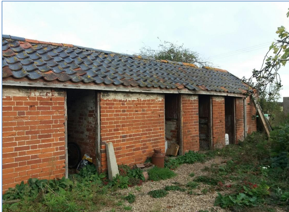
Diminutive historic outbuilding constructed in monk bond brickwork – traditional but less common than other bonds. The building also features both black glazed and red clay pantiles on its roof, and clay hogs back ridge tiles which are also very characteristic.
