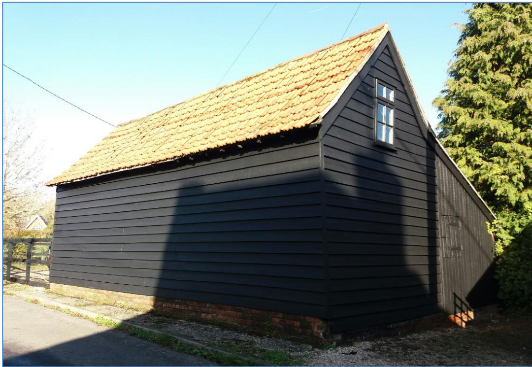
Weatherboarded outbuilding which references an agricultural aesthetic.
