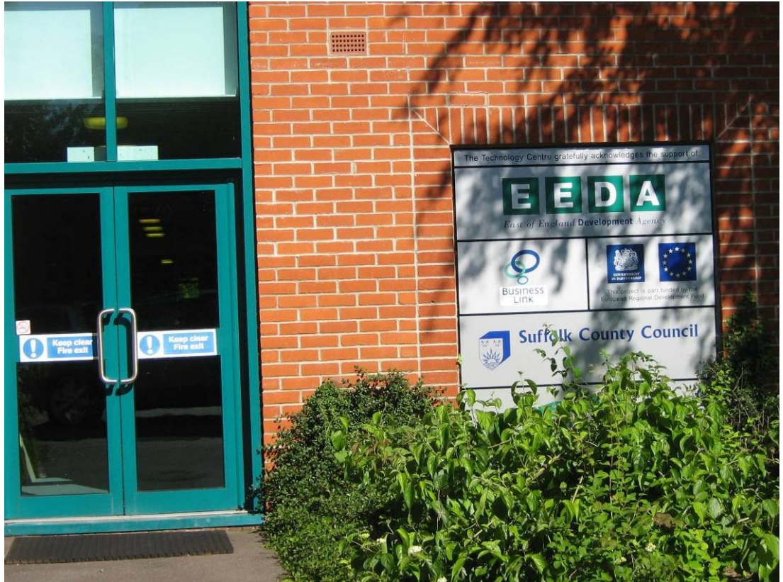
Figure 5 Framlingham Technology Centre, Framlingham
