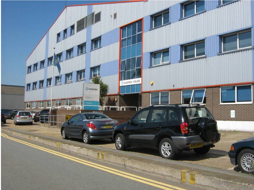
Figure 2 Maersk Office, Felixstowe Port
