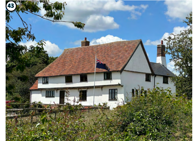
Plate 23 Hubbard's Hall, grade II listed building dating to the 16th century.
