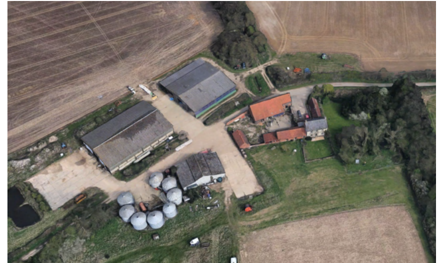
Figure 23 Grove Farm, showing historic ancillary structures with red brick roofs, and much larger modern agricultural sheds to the west.
