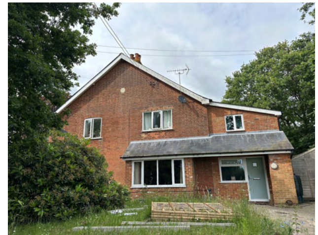
Plate 50 Inappropriate plastic windows and altered fenestration to 5 Potash Lane.
