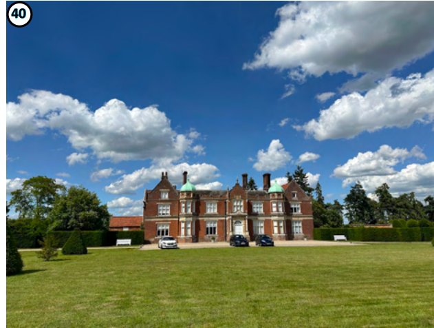
Plate 22 Bentley Manor, a late 18th century structure featuring significant Victorian alterations and extensions.
