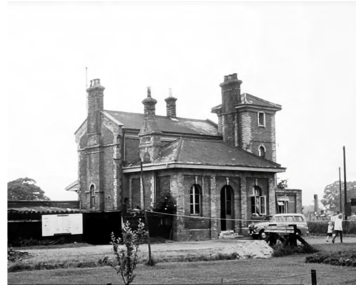
Figure 10 Undated photograph showing Capel Station's northern elevation.
