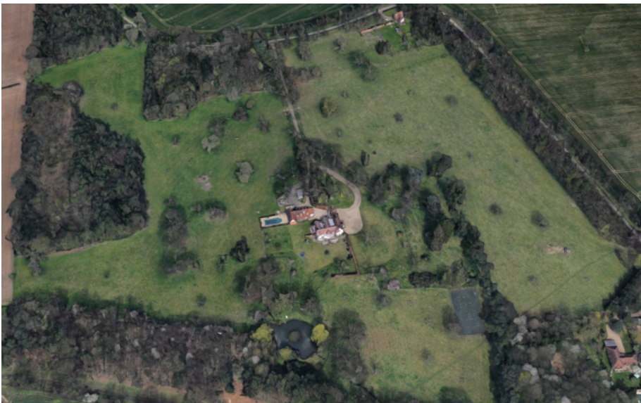
Figure 21 Bentley Park showing principal dwelling and ancillary structures. The site still retains much historic park land, ancient wood and long driveway.
