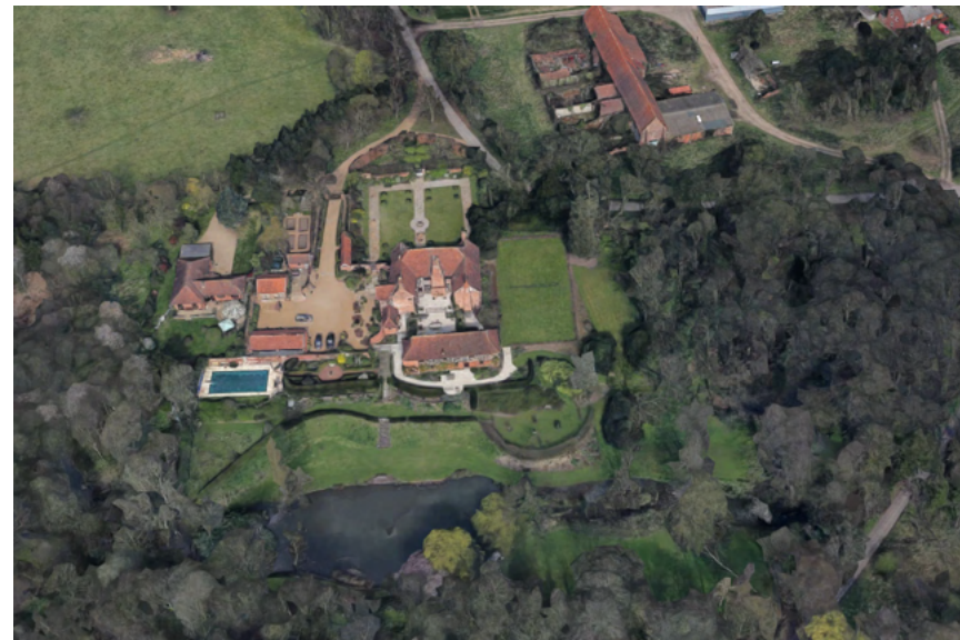
Figure 19 Bentley Hall showing formal gardens, numerous ancillary structures, fishponds and highly wooded setting.
