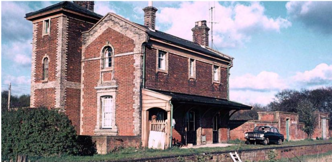
Figure 9 Undated photograph showing Capel Station's southern elevation.
