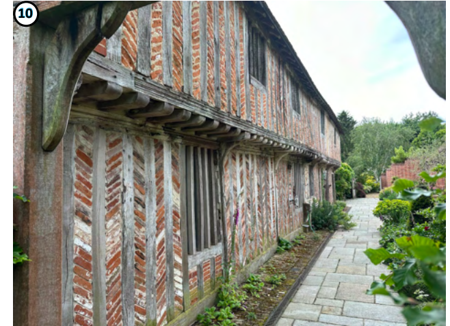
Plate 11 Bentley Hall Stables/Meeting Hall showing herringbone brickwork and closely spaced joists.
